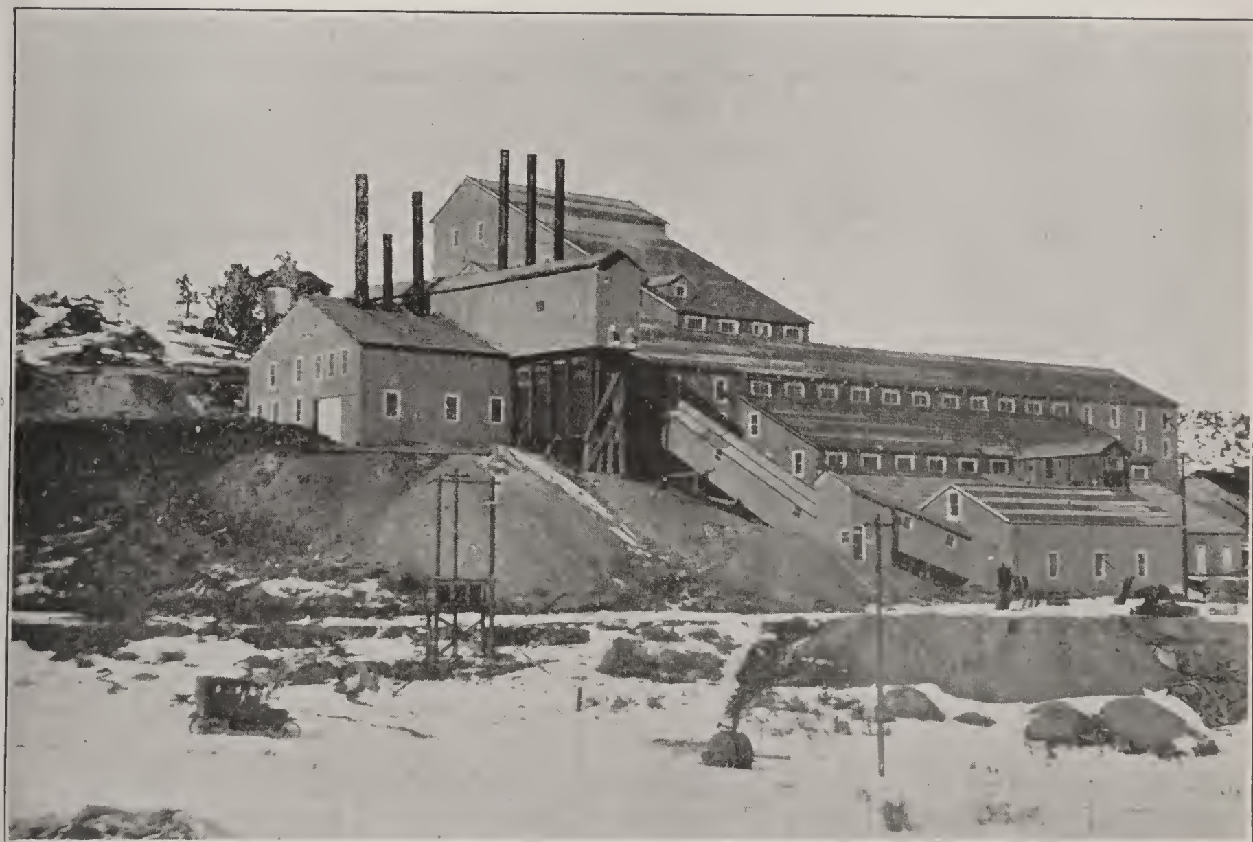
Pneumatic Flotation Plant
