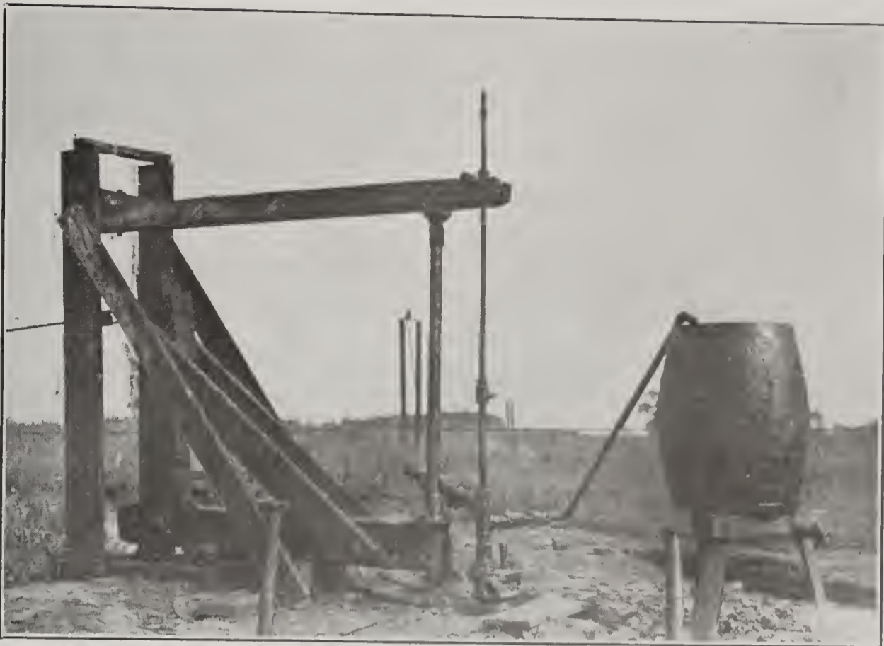
Fig. 24. Photograph of a single-barrel gage setup used early in the work.
