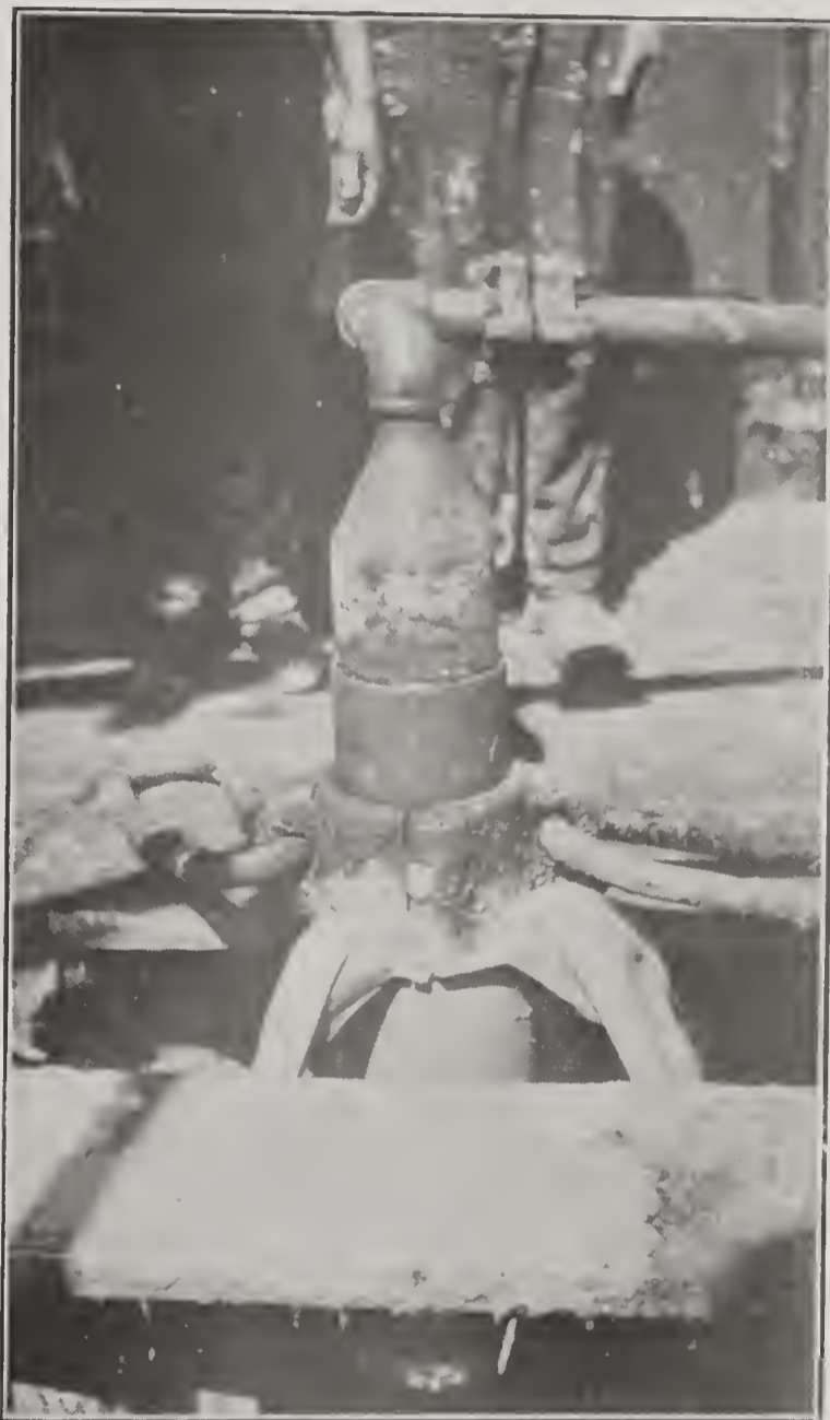
Fig. 32. Photograph showing the connection at the top of the well between the discharge of the mud pump and the casing in the circulation method. The outgoing mud fluid has been down through the casing, out its bottom, and is returning to the surface, outside the casing.
