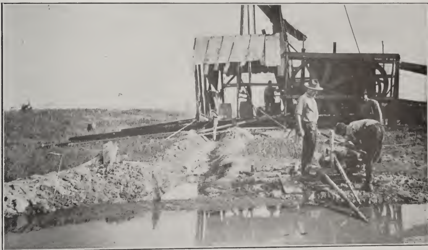
Fig. 35. Photograph of the mud sump looking toward the derrick. Trench near the center in which coarse material settles out; suction and mixing pipes at the right, the former below the latter.
