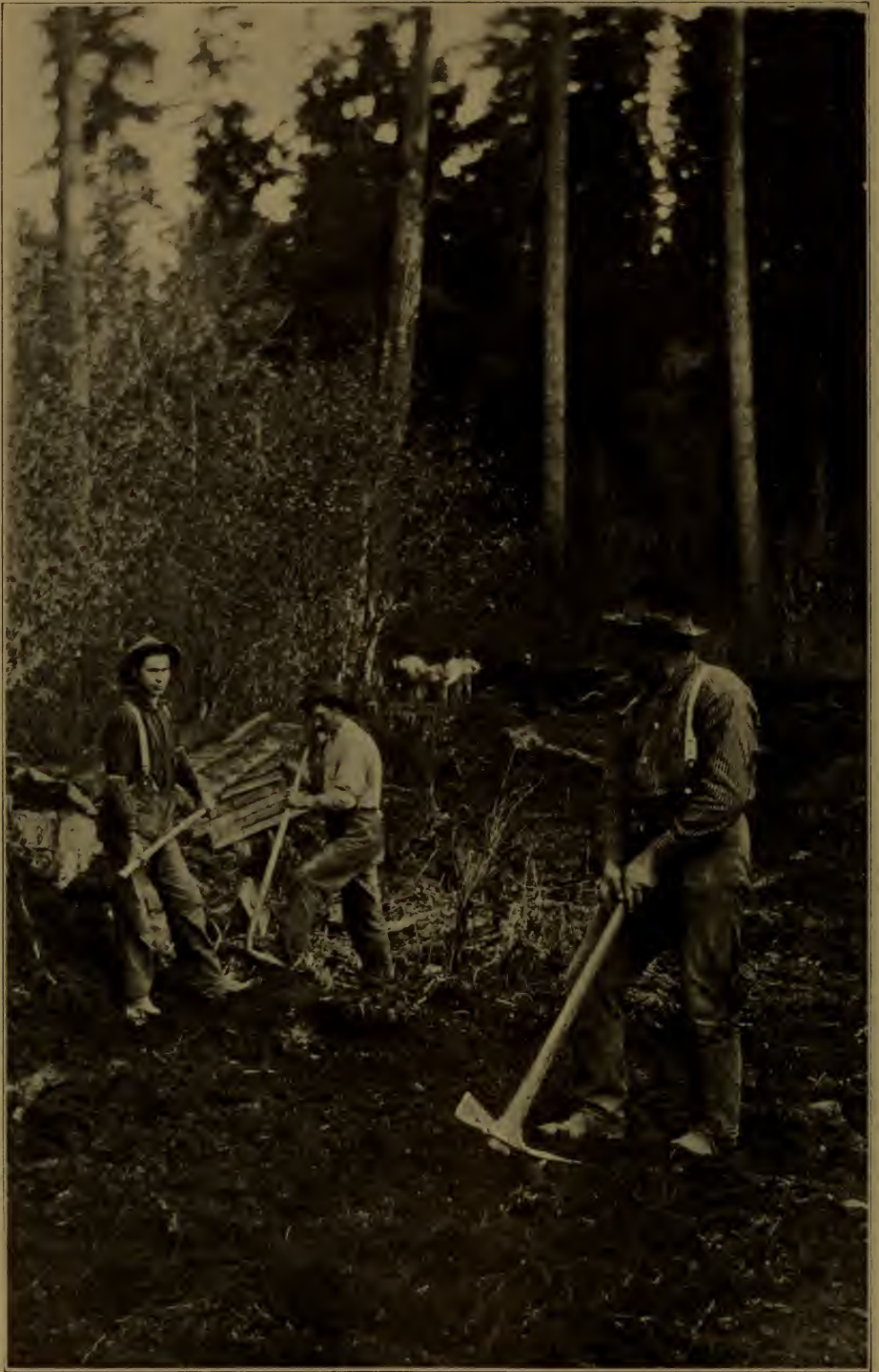
Workers on the road.
