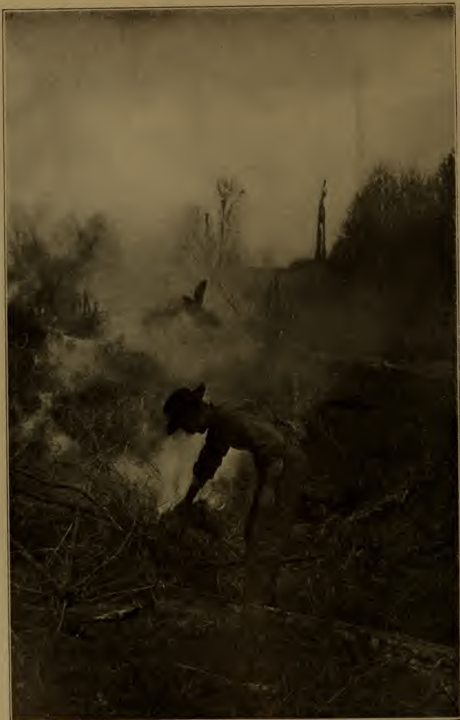
Clearing the land.
