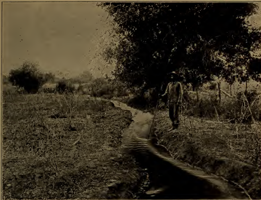
The ditch carrying water from main supply.
