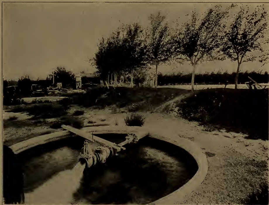
Artesian well with a water flow coming from 1,600 feet beneath the earth's surface.
