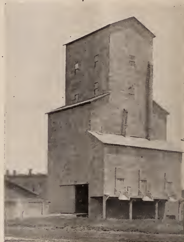
PLANT OF THE FARMERS GRAIN COMPANY, LATHAM, ILL.
