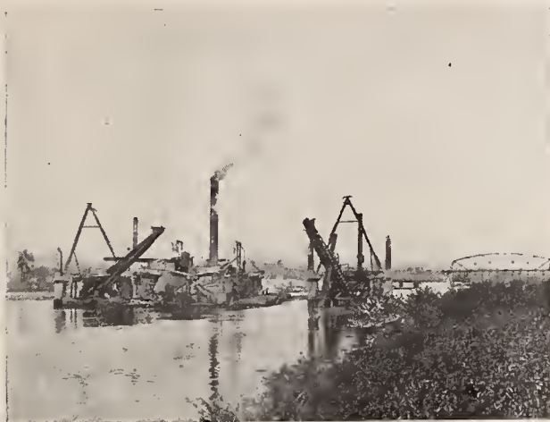
DREDGING OPERATIONS IN THE NEW CANAL
