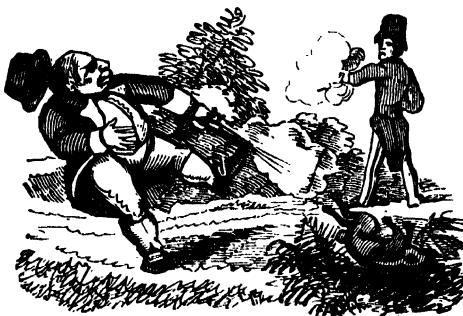
EXCHANGING—RECOVERING THE DIFFERENCE.
