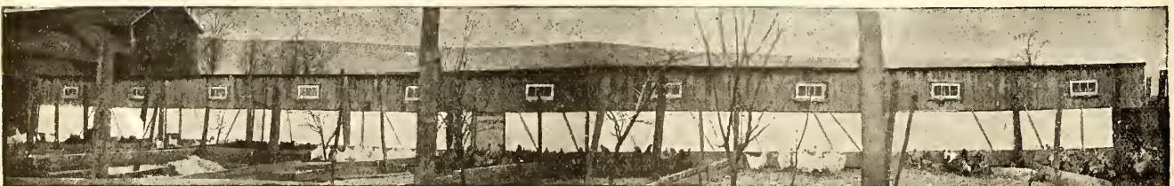
The above illustration is the one referred to by Mr. Howell as a muslin front house. Note how the muslin is placed; this is somewhat different than in the majority of houses of this type
