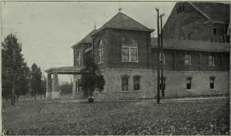
PRESENT GYMNASIUM. New building now being erected.
