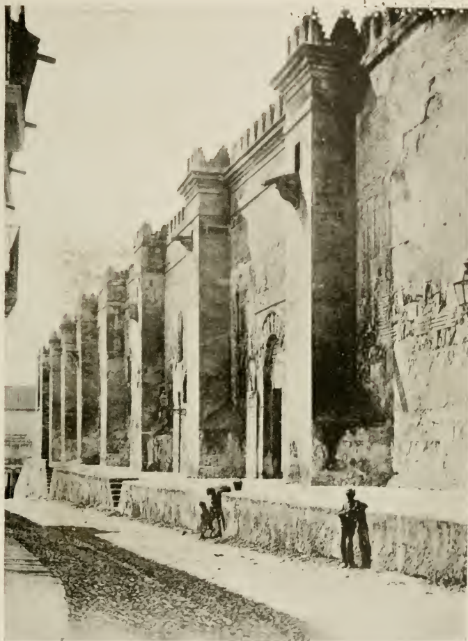
EASTERN FAÇADE OF THE MOSQUE.
