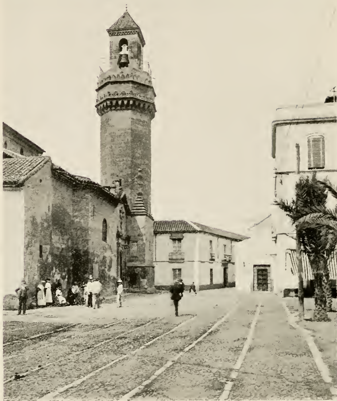
ANCIENT ARAB TOWER, NOW THE CHURCH OF ST NICHOLAS DE LA VILLA.
