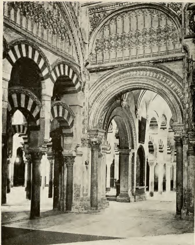
INTERIOR OF THE MOSQUE.
