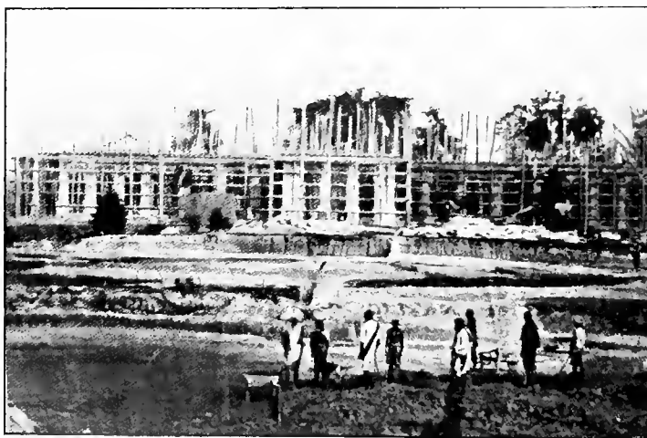
GOVERNMENT HOUSE GARDEN BEING LAID OUT BY CONVICTS.
