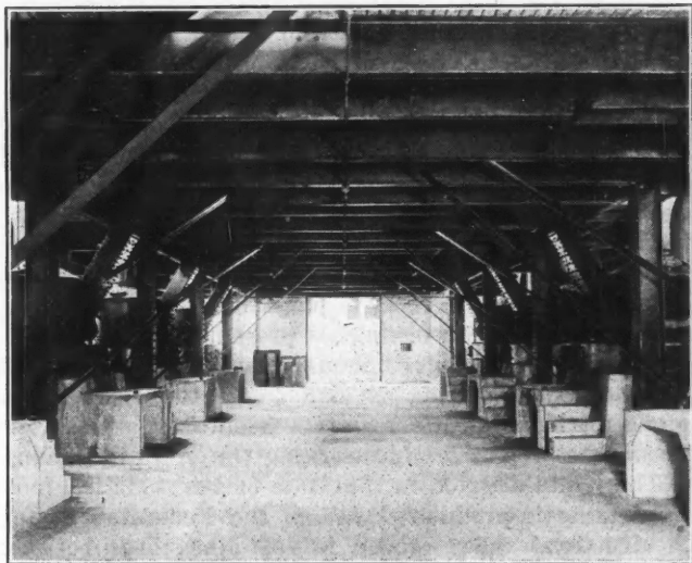
FIG. 3. THE PULVERIZER MILL BUILDING. MAIN AISLE
