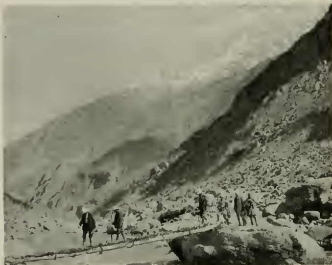
TEMPORARY BRIDGE OVER THE BRALDOH BELOW CHONGO.
