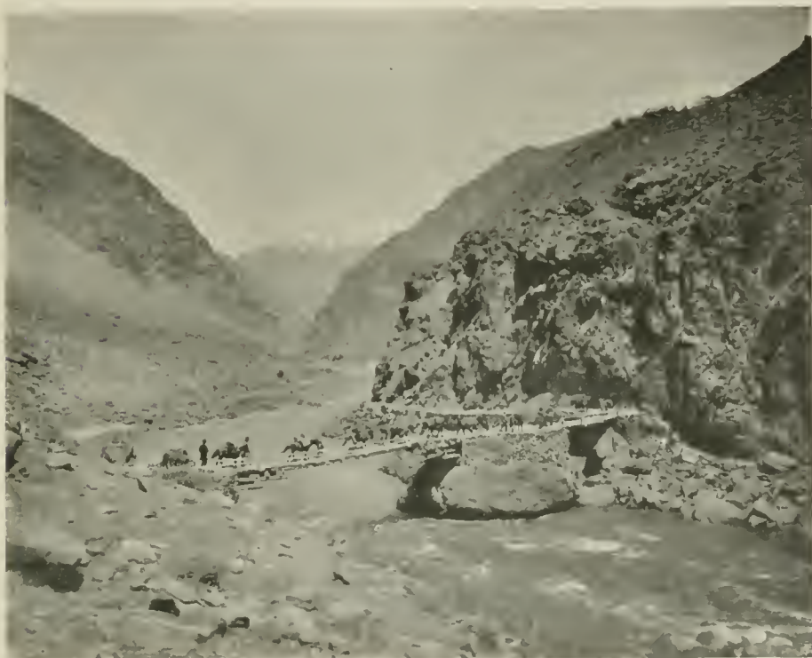
CANTILEVER BRIDGE OVER THE DRAS.
