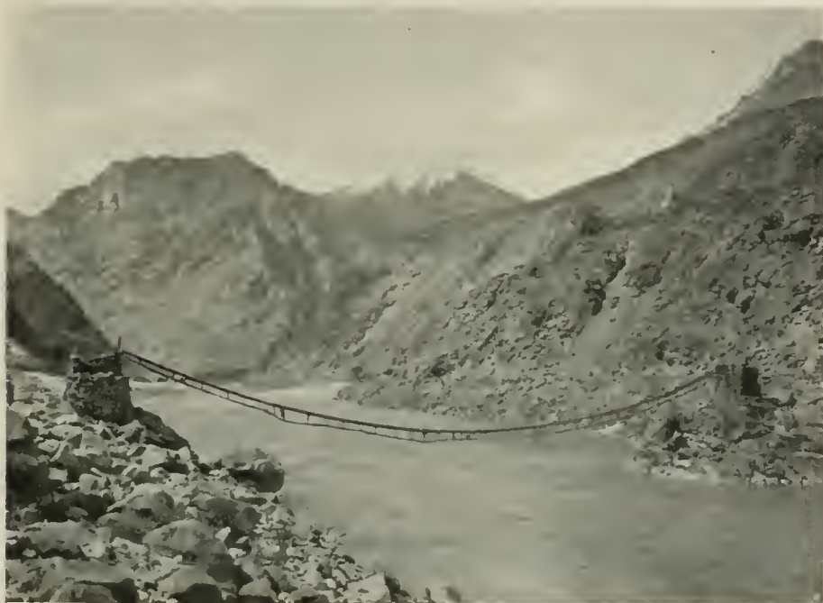
JHULA BRIDGE AT KARMANG.
