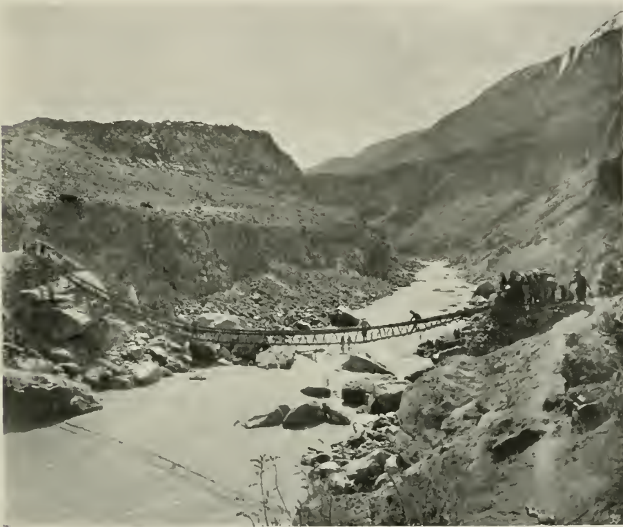
ROPE BRIDGE BETWEEN PAKORA AND CHONGO.
