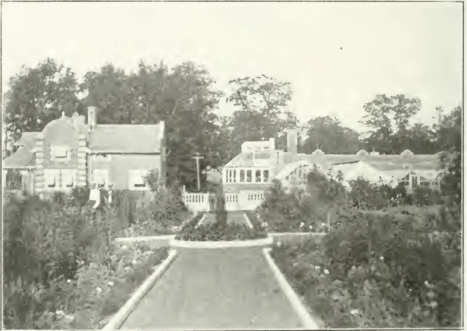
Cement Curbs used to good advantage. Photo from Sir H. Pellatt.
