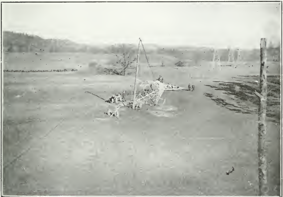
Erection of Standard Tower, Dundas Valley.
