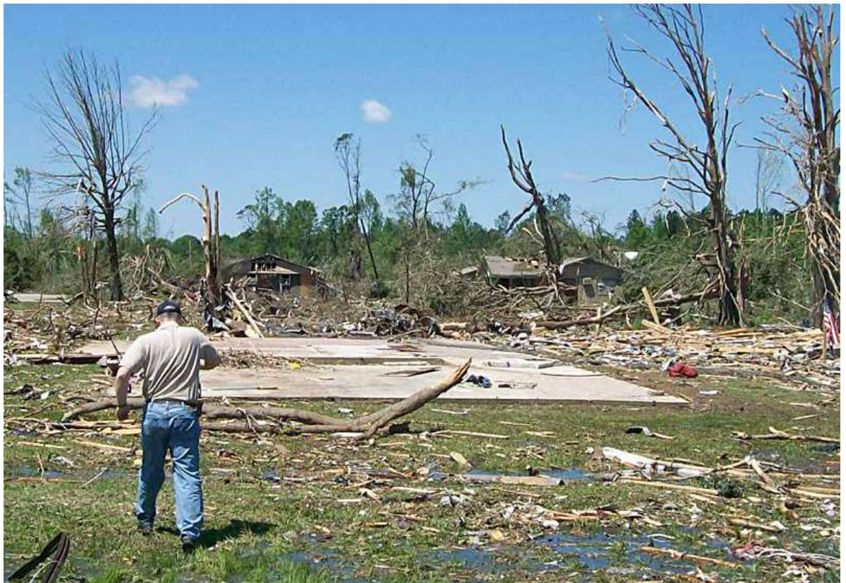
Slab wiped clean with only anchor bolts protruding from perimeter of slab. One fatality and two serious injuries at this location. Hardwood tree in background debarked. Rich Okulski, Warning coordination Meteorologist (WFO Memphis) surveying damage. Photo location one mile west of Smithville, MS. (Photo: WFO Memphis)
