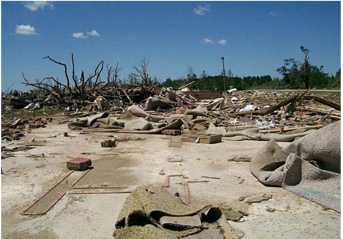
Looking north, a slab with no standing walls. Debarked hardwood trees in background. Photo location Smithville, MS. (Photo: WFO Memphis)
