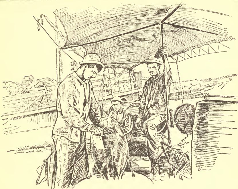
ADJUSTING MOTOR MECHANISM OF A TORPEDO.
