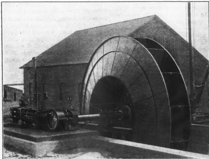
35-FT. FAN, WITH TAPER BLADES, CONNECTED TO REYNOLDS-CORLISS ENGINE
