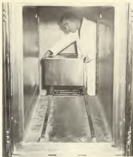
Delivering media by autoclave from central services to pilot plant.
