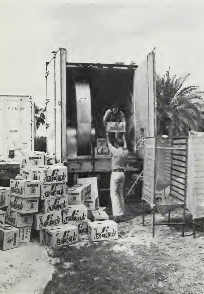
Research entomologist Donald L. von Windeguth and research assistant Frank Cavaliere load infested grapefruit into an experimental fumigation chamber (1174X1737-20).
