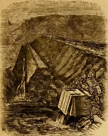
Fig. 1.—TIDE GATE AND DIKE.
