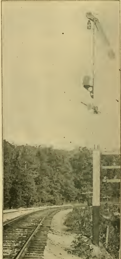
Home Signal "Cleared."
