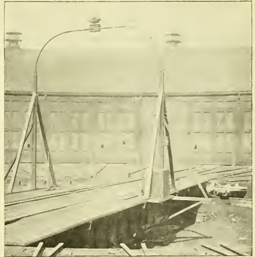
Electric Motor Driving a Turntable.
