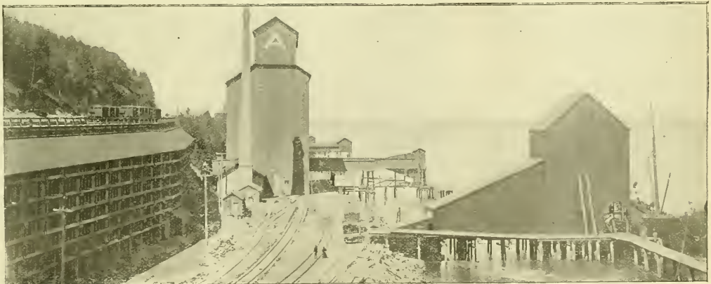
General View of Bunker and Chute Tower.
