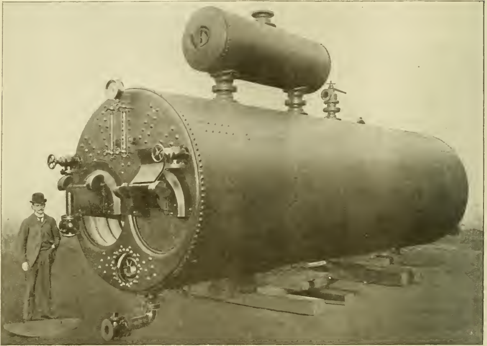
A Lancashire Boiler with Welded Shell.—Built by the Continental Iron Works.
