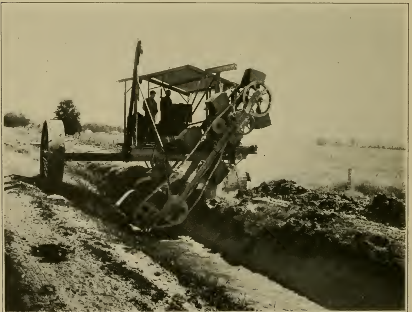
2. CLEANING AN IRRIGATING DITCH WHILE IN OPERATION.
