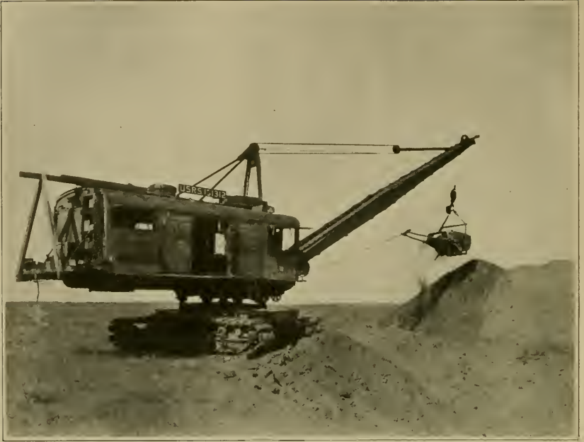
1. EXCAVATION BY DRAG LINE.
