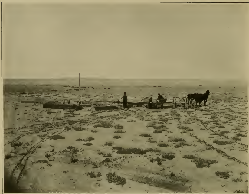
1. THE NEW HOME BEING STARTED.
