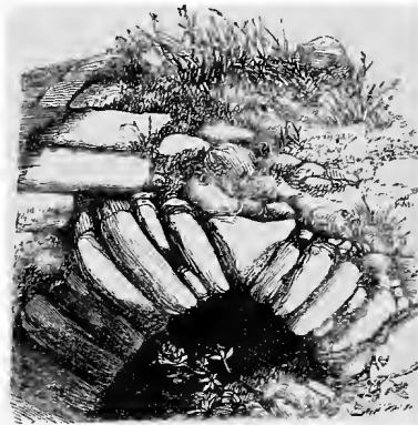
Fig. 9. Exposed section of the arch of the vault.
