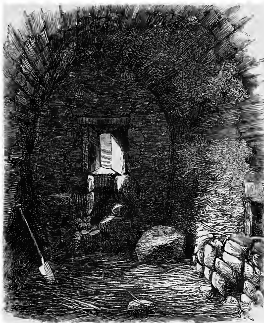
Fig. 8. Interior of the building, showing splayed window in eastern gable, recess in interior of south wall, vaulted roof, etc.
