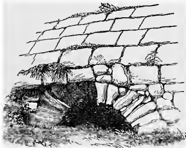
Fig. 6. Semi-circular arch of the door as seen from without, the garden earth filling the doorway.
