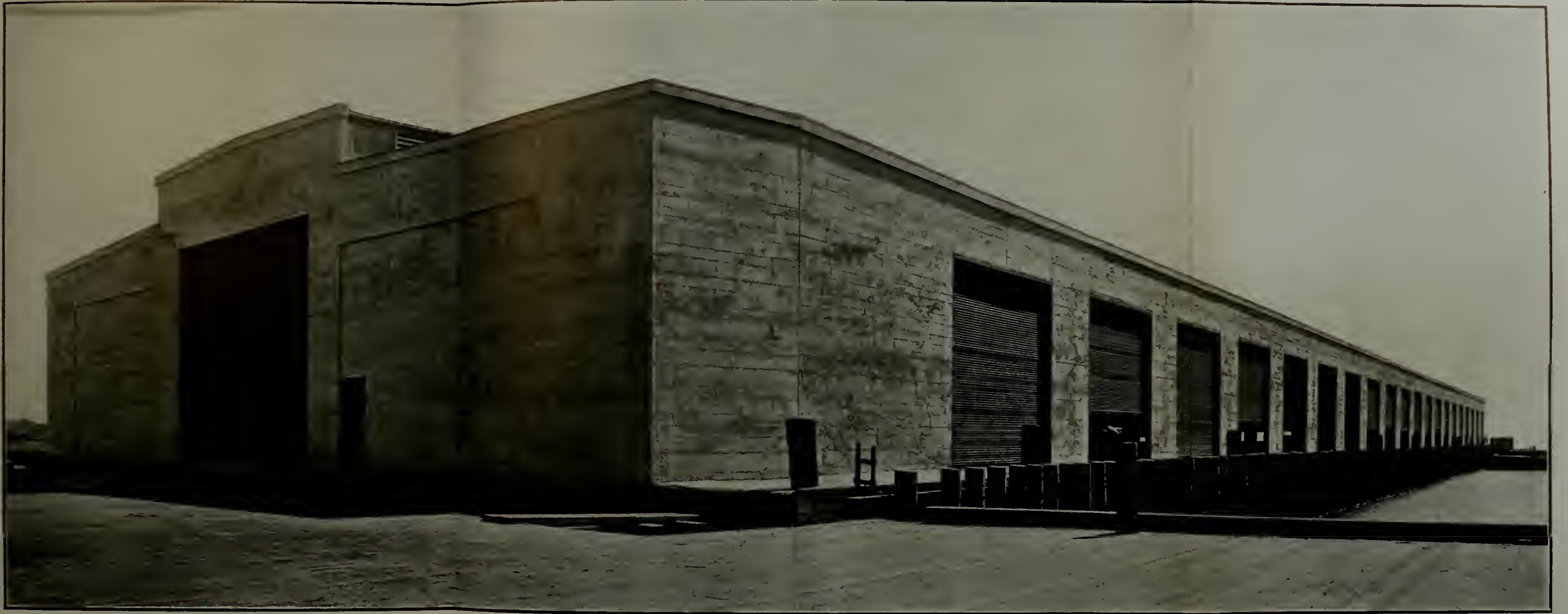
PIER 40, SHOWING TYPE OF REINFORCED CONCRETE SHED.
