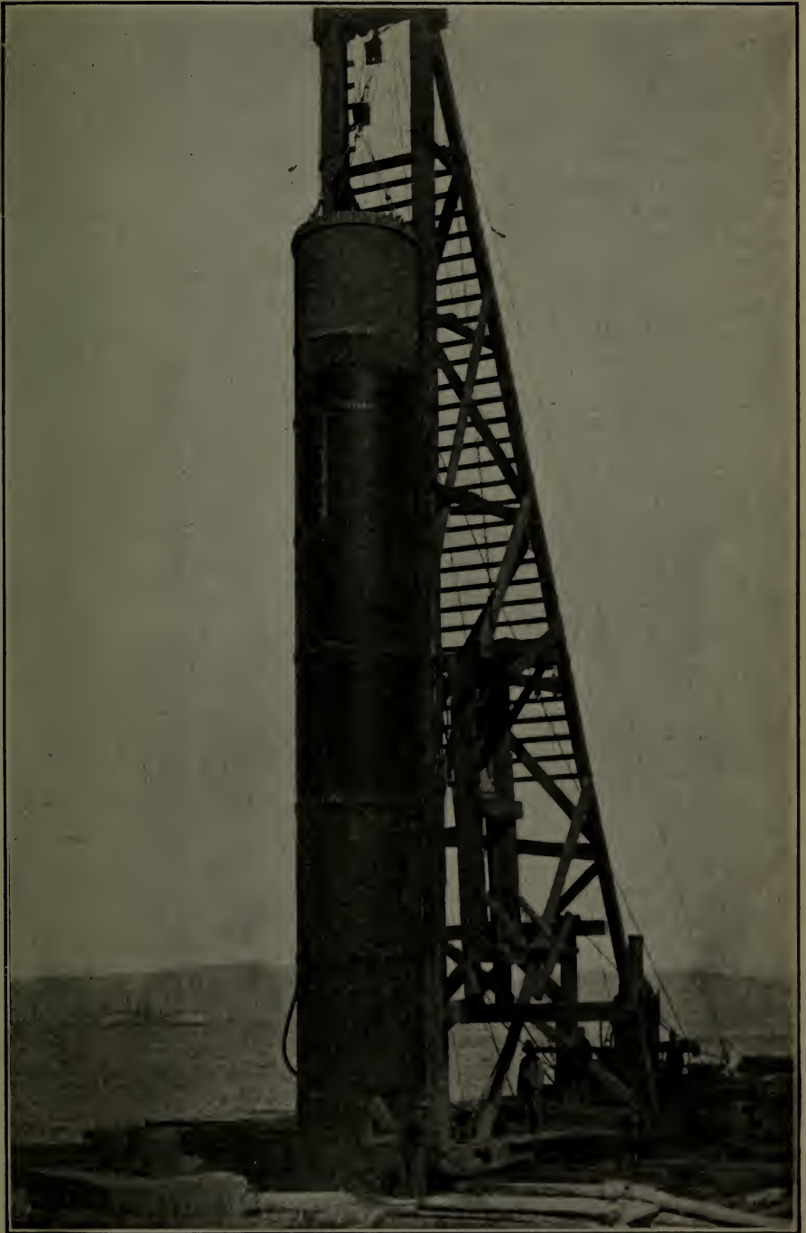
Steel cylinder for concrete pillars of new piers.
