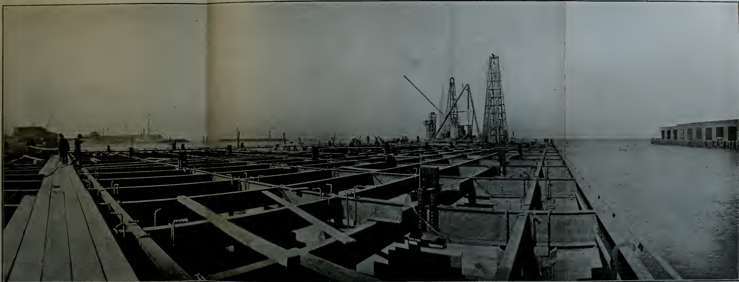
PIER 38 IN COURSE OF CONSTRUCTION, SHOWING STEEL FLOOR BEAMS AND GIRDERS.
