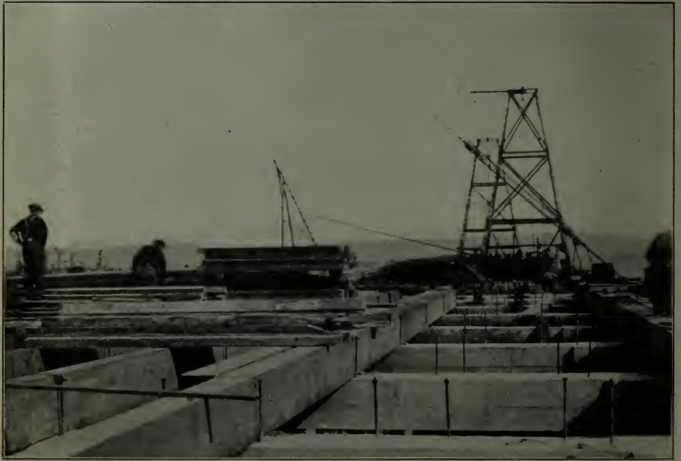
Concreted steel beams of pier 34.
