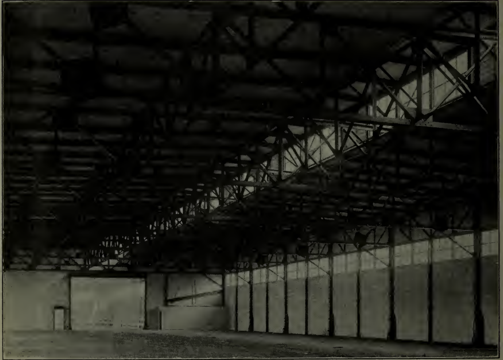
Interior of steel shed on new pier No. 36.
