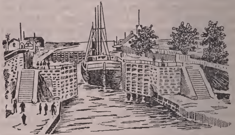
LIFT LOCK CANAL.
