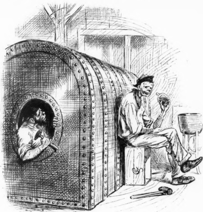
IN THE BOILER SHOP.
