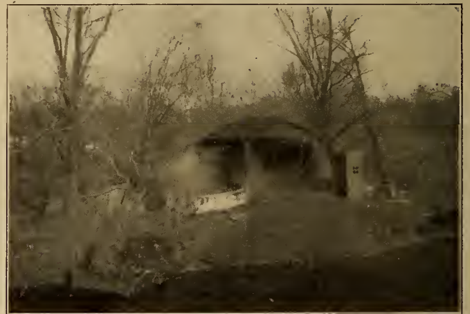
Dynamiting the bridge.
