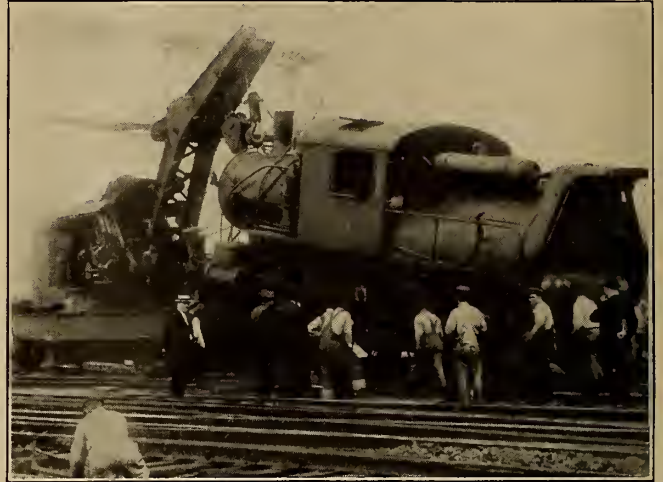
Replacing locomotive on its tracks after a wreck in yards of Central Railroad of New Jersey. Copyright, 1915, by Pathe News.
