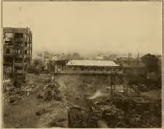
A reconstruction gang was at work in the Edison plant within a few hours after the last fireman departed from the scene.
