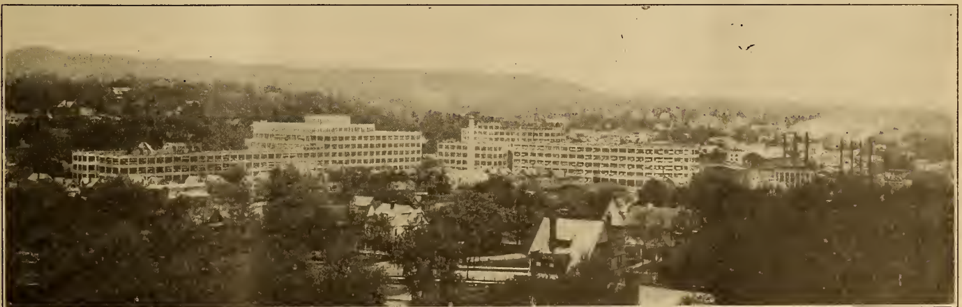
A general panoramic view of the Edison plant at Orange, New Jersey, before the recent fire.
