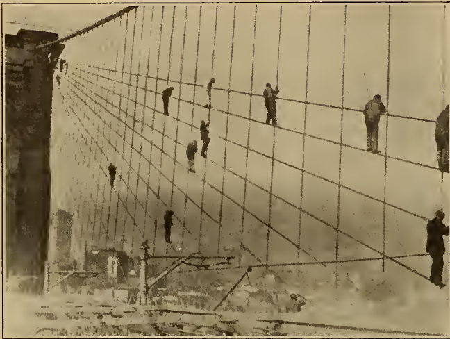
Painters at work on the Brooklyn Bridge high above the river. Copyright, 1914, by Hearst-Selig News Pictorial.
