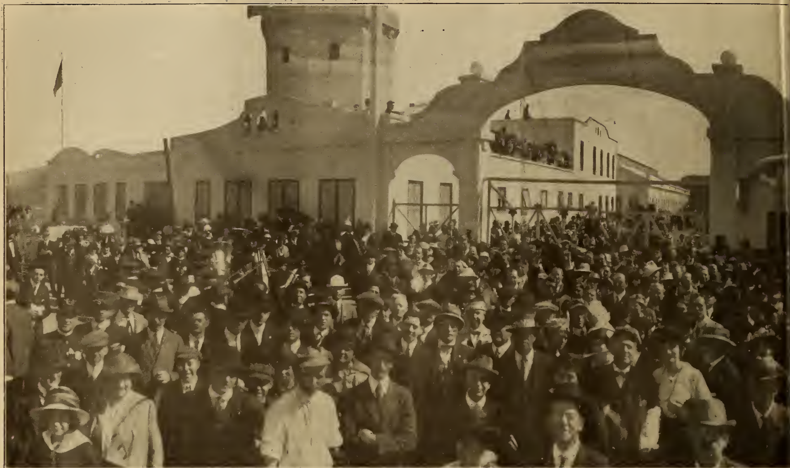
This photograph was taken March 15, 1915, just prior to the official opening of Universal City.
