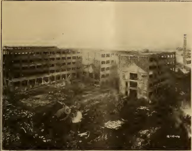
A portion of the Edison plant taken the morning after the fire.
