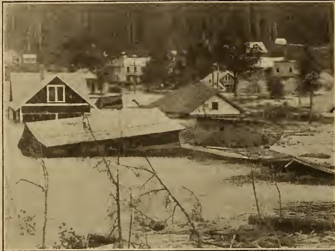
Great damage done by floods at Cedar Falls, Wash. Copyright, 1915, by Pathe News.
