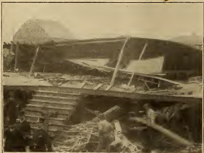
Wreckage of orphanage at New Orleans, Louisiana. Copyright 1915 by Pathe News.
