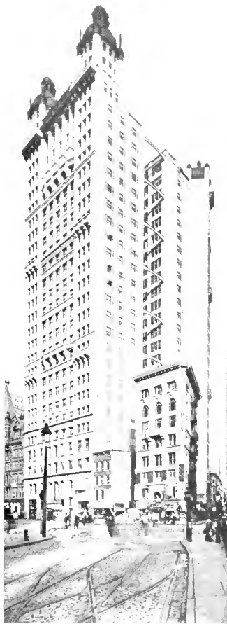
Park Row Building , at No. 13-21 Park Row, overlooking the Post Office. 31 stories, 390 feet high to top of towers. Foundation is sunk 75 feet below the street level. Total cost of building and land, $4,000,000.
