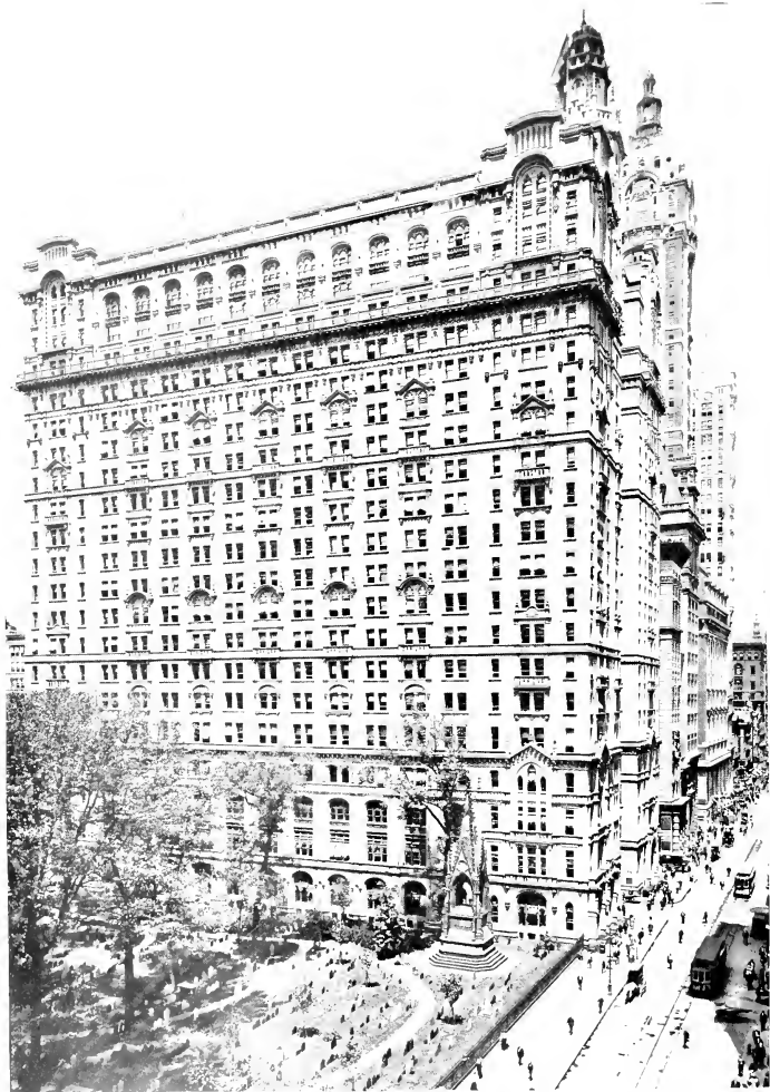
Trinity Building, at 111 Broadway, overlooking Trinity Church and abutting the U. S. Realty Building, with which it is connected. Each building is 4 stories, 330 feet high, and the value of the combined buildings is $15,000,000. The foundation consists of 70 pneumatic caissons, each one sink 80 feet below the sidewalk. Copyright, 1908, G. P. Hall & Son, N. Y.
