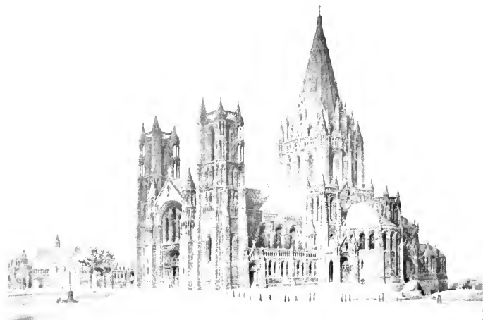
Cathedral of St. John, the Divine. At 111th Street, near Morningside Park. The most important Protestant Episcopal Church in America. Construction began 1892, consecrated April 19, 1911. Cost $3,500,000, several million dollars more required for completion.
