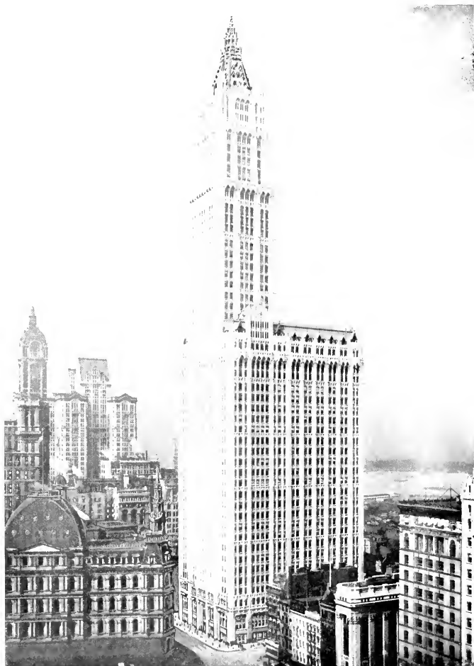
Woolworth Building. Bounded by Barclay Street to Park Place. Tallest office building in the world; 55 stories; 291½ feet high, including spire, $14,000,000; plot 132 x 197 feet. Foundation consists of caissons 19 feet in diameter sunk 110 to 130 feet. The 24th floor contains the executive offices of the F. W. Woolworth Co., largest 5 and 10 cent syndicate in the world, operating over 700 stores.
