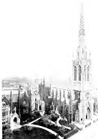
Grace Church —Protestant Episcopal, at Broadway and Ninth Street. Built 1845, of white limestone, with marble spire. James Renwick, architect.
