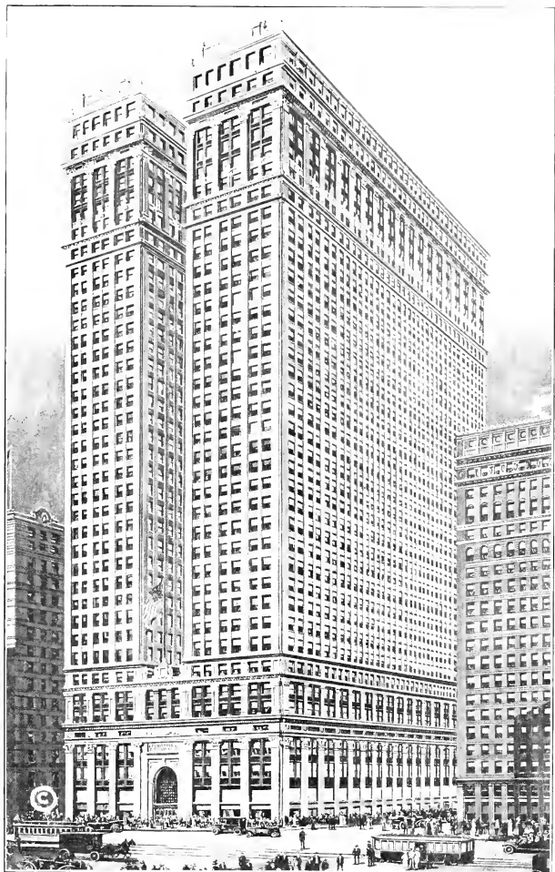
Equitable Building. built on the site of the old Equitable Building, which was destroyed by fire on January 9, 1912. It is a 38-story office building, 537.6 feet above the street level, covering an entire square block, with a floor area of nearly 45 acres. It will be a city of 15,000 workers. The building and land cost $29,000,000. Copyright, 1913, by the Equitable Building Corporation, N. Y.
