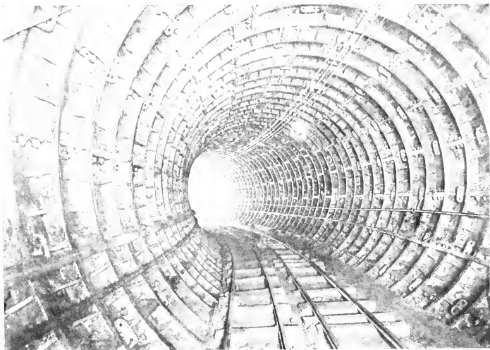
Hudson River Tunnel, built by the Hudson and Manhattan Railroad System. Construction started Sept., 1874. Officially opened Feb. 25, 1908. Two single track tubes, with a minimum inside diameter of 15.3 feet. Approximately 5,700 feet long.
