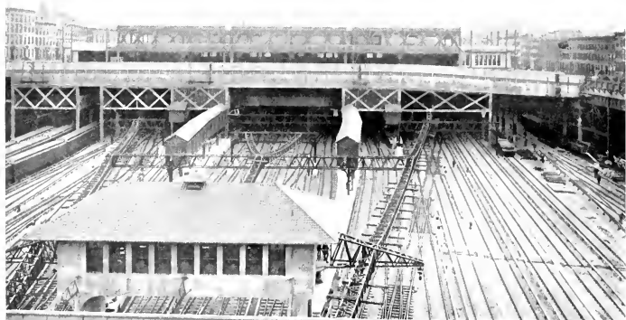
Trackway of Pennsylvania Railroad. Running from the great Depot at Seventh Avenue through six tunnels under the Hudson River. The bed of the tracks in midstream is 100 feet below the river. A bridge extends over the tracks from 31st to 33rd Streets, with stairways leading down to the tracks. The New Post Office is built over these tracks at Eighth Avenue.
