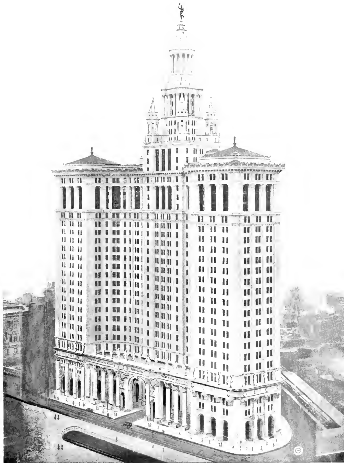
The New Municipal Building , on Park Row, facing City Hall Park, completed in 1913. It contains offices for the various city departments, which are now paying a rental of over half a million dollars yearly. It is a 34-story structure, 539 feet above the sidewalk. The foundation, the most difficult ever attempted, is 130 feet deep, of which 90 feet is below the water level. The floor area is 699,000 square feet. Total cost, $12,000,000.
