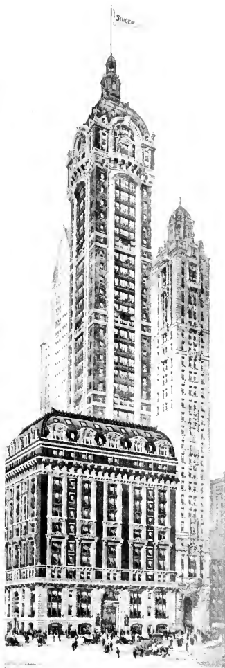
Singer Building at Broadway and Liberty Street, 29 stories, 612 feet high above the sidewalk, 724 feet from basement floor to top of flagstaff. 9½ acres floor space, total weight, over 18,000 tons. Supported upon an edifice of solid concrete, sunk 92 feet below the curb.
