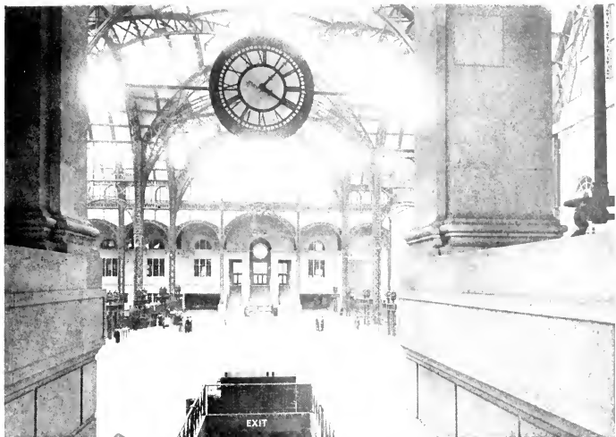
Interior of Pennsylvania Railroad Station. The main concourse, in imposing room of white marble, 40 x 210 feet, extends under the street. Two stairways lead to each train platform. The exit concourse is 60 x 100 feet, and elevators carry passengers from there to trains.
