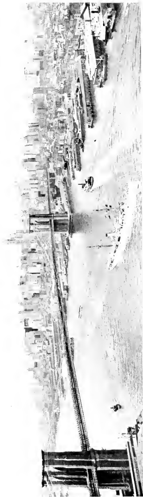
Brooklyn Bridge. Running over the East River from Park Row, in Manhattan, to South Street, Brooklyn. Construction was begun in 1876, and the bridge was opened to traffic in 1883, having cost $24,000,000. The total length of the bridge is 6,337 feet, and the width 85 feet. The towers are 228 feet high above water level, while the clear height at center of span is 135 feet above the water. Copyright, 1908, G. P. Hill & Son, N. Y.
