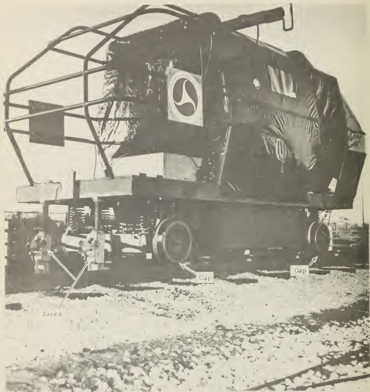
Vehicle in Jacked Position
