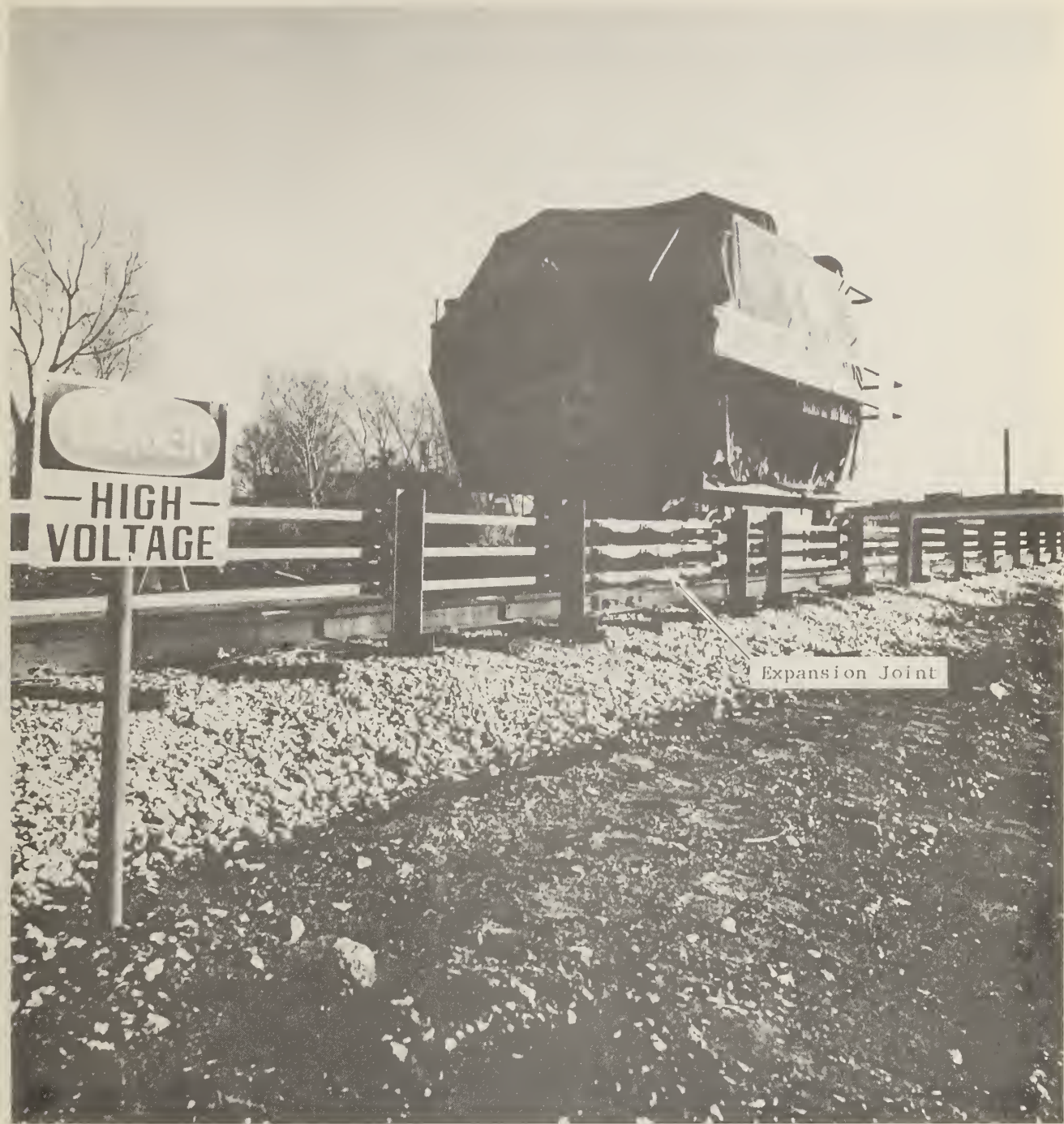
Expansion Joint - Power Rail
