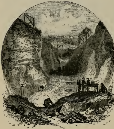
ENTRANCE TO BALTIMORE TUNNEL.
