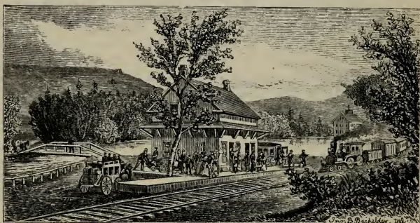
RAILROAD STATION, BETHLEHEM, N.H. Boston, Concord, and Montreal R.R.
