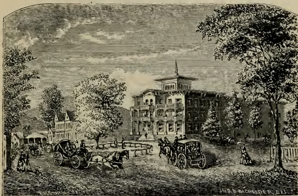
LANCASTER HOUSE, Lancaster, N.H.
