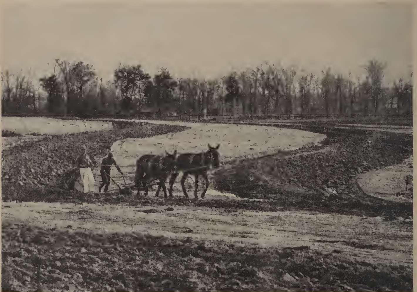
PLATE 11.—Illustration of terrace construction with plow and mule power; this can be done by any farmer when terracing machinery is not available.
