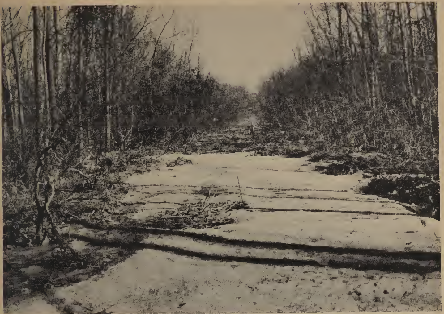
PLATE 6. Channels plugged with sand and debris cause swamping on adjacent flood plains.
