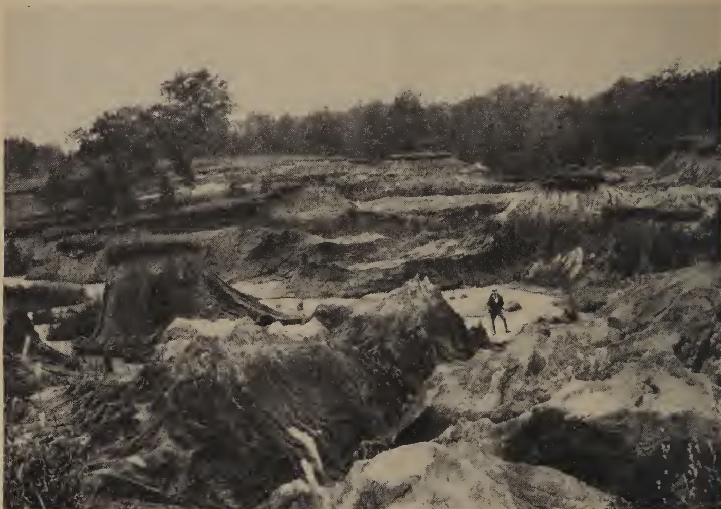
PLATE 8.—Abandoned upland area in the Brown Loam; it is severely gullied and completely destroyed for further agricultural use.
