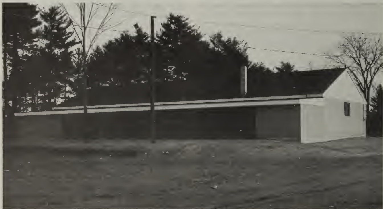
Combination Shelter, Concession Stand, Outdoor Restrooms
