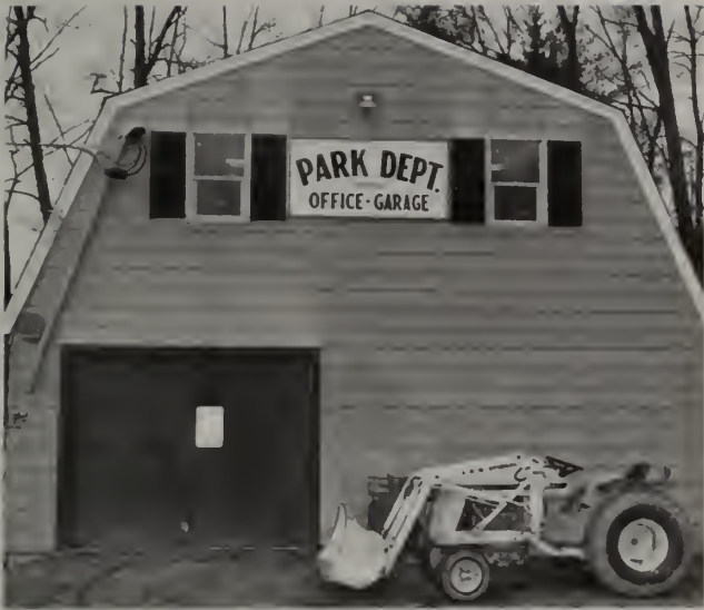
Park Garage and Office
