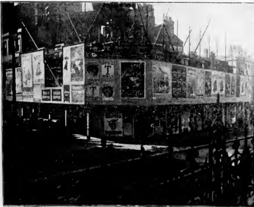
Hoarding around the site for the Pearl Life Assurance Co.'s new building. St. John's Street, near St. George's Hall, Liverpool.
