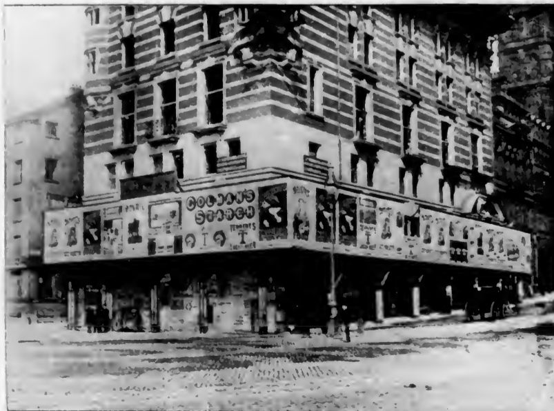
Another Liverpool Hoarding. The White Star Steamship Co.'s Building, St. James St.
