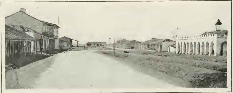
Port of Casilda, Santa Clara Province and macadam road connecting it with Trinidad.
