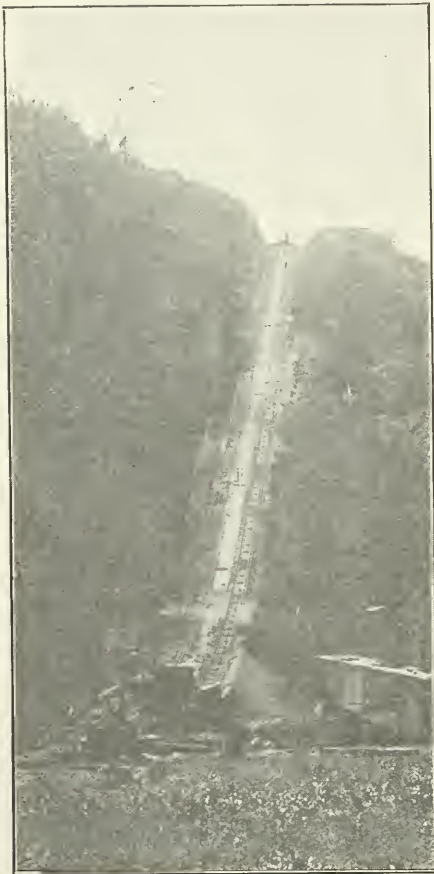
Inclined railway for the removal of iron ore to the coast from the mines of the Spanish-American Company at Daiquiri.
