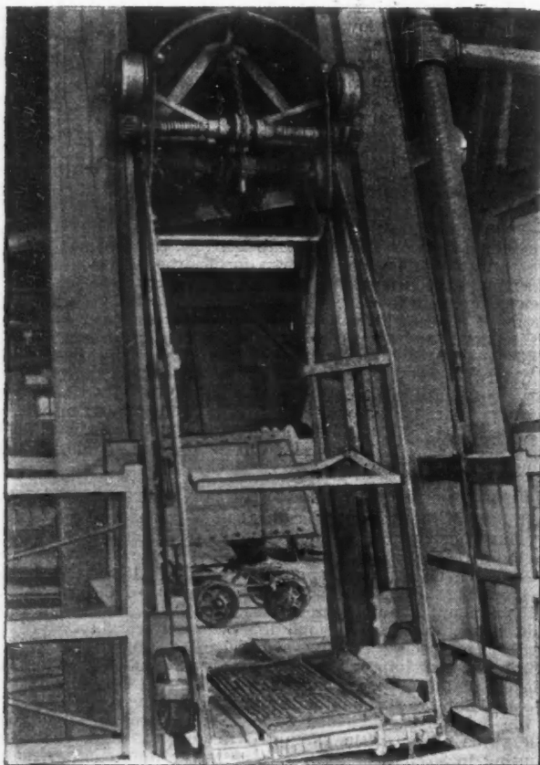
CAGE FOR INCLINED SHAFT AT ORIGINAL MINE, MONTANA.
