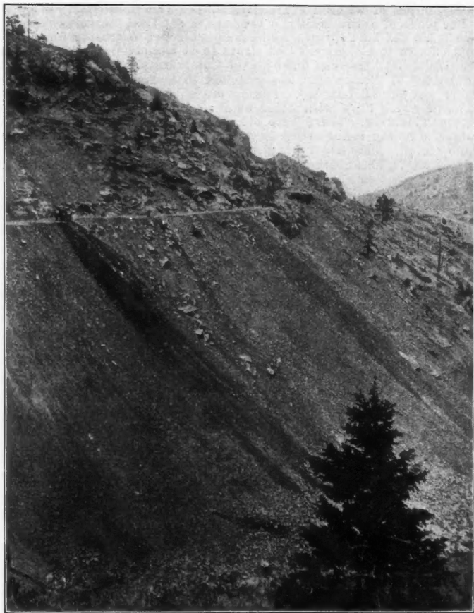
SIDE HILL CUT, COLORADO SPRINGS & CRIPPLE CREEK RAILROAD.
