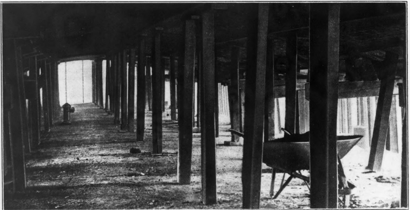
REVERBERATORY FURNACE WITH SIDE WALLS REMOVED
