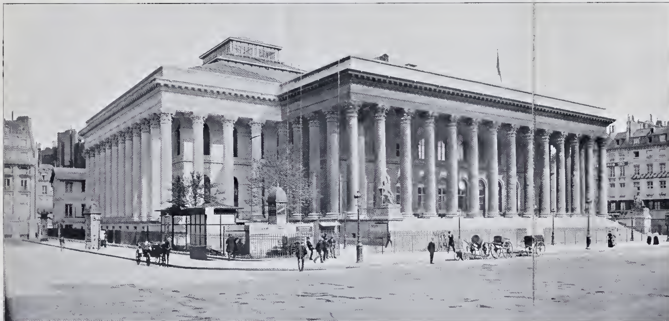
THE BOURSE, PARIS. SHEWING THE RECENT ADDITIONS.—M. CAVEL, ARCHITECT
