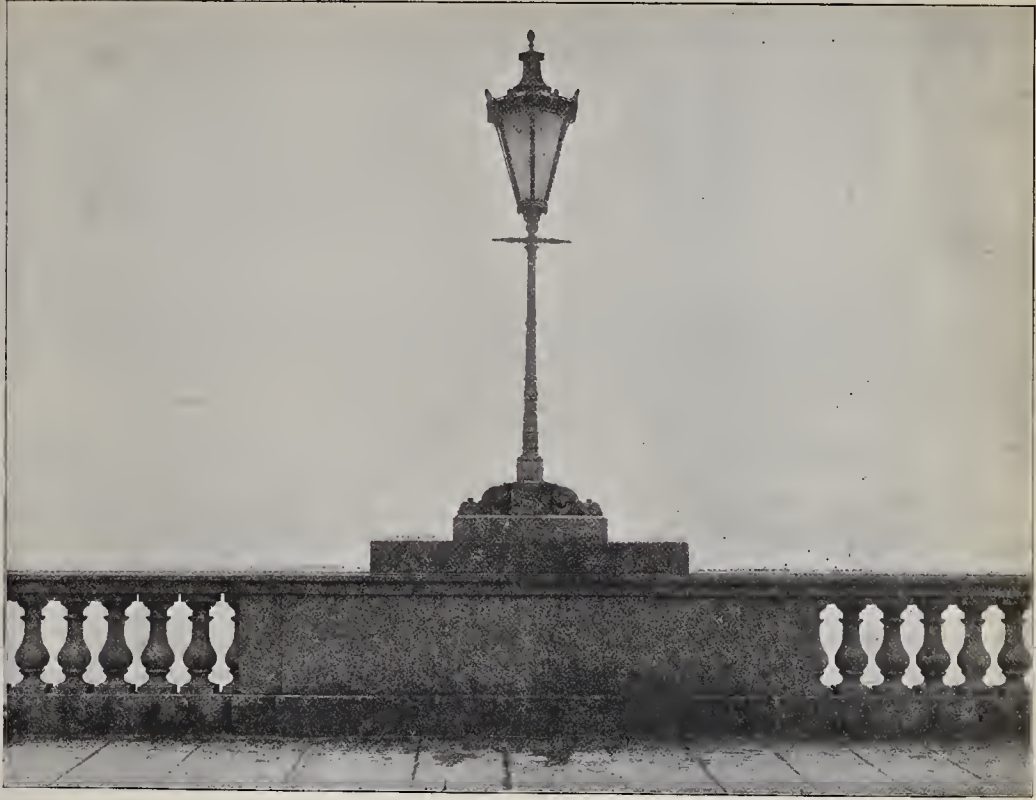
New Lamp-standard, Waterloo bridge. From a Photograph.
