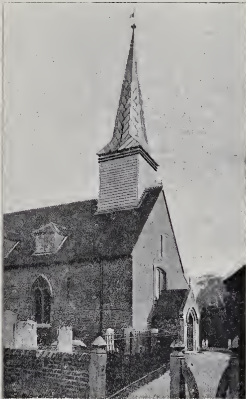
Fig. 4. Chipping Ongar Church : North-west View.
