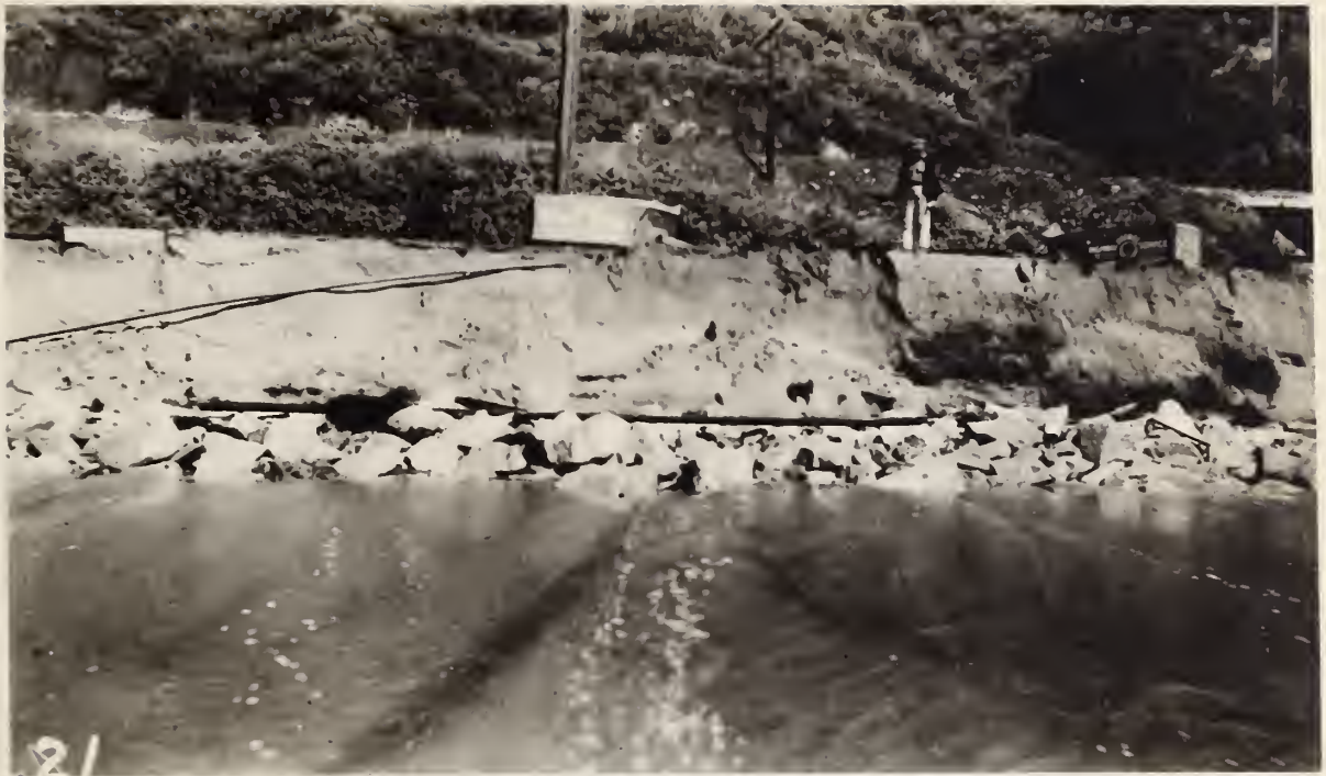
FIGURE 4. - 30-FOOT CRUSHED ROCK ROADWAY ON A SAND FILL BUILT BY THE STATE ON THE MIDDLE SECTION. PICTURE TAKEN BEFORE FILL HAD BEEN WASHED AWAY.
