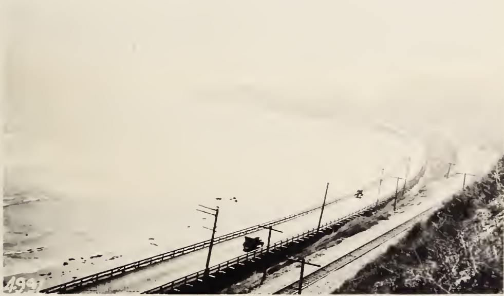
FIGURE 2. - BIRD'S-EYE VIEW OF THE OLD TIMBER-TRESTLE CAUSEWAY ON THE NORTHERLY END OF THE PROJECT.
