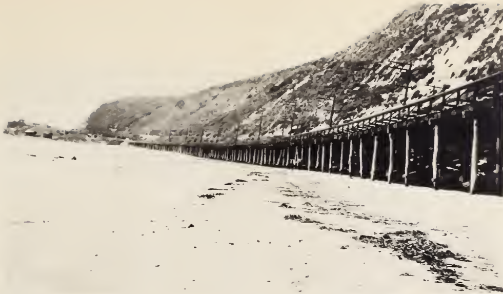
FIGURE 1. - OLD TIMBER-TRESTLE CAUSEWAY ON THE NORTHERLY SECTION OF THE PROJECT.
