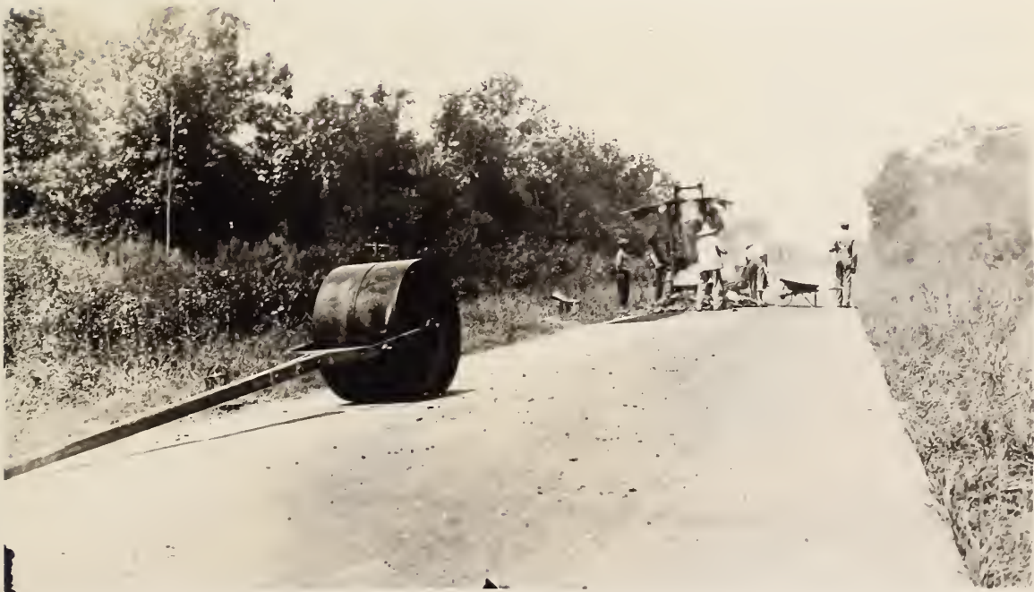
FIGURE 2. - HAND ROLLER. REPAIR GANG AT WORK AND PORTABLE PLANT IN BACKGROUND.
