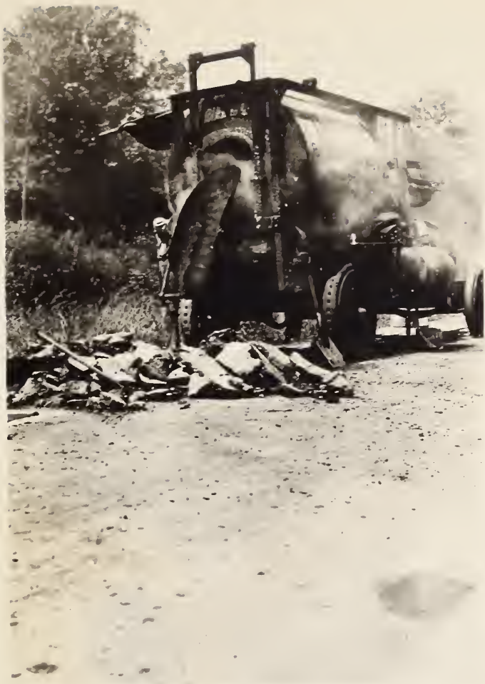
FIGURE 1. - SALVAGED BITUMINOUS SURFACING MATERIAL READY FOR CHARGING PORTABLE PLANT.
