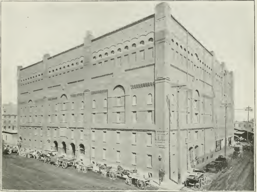
FIG. 1.—RICHMOND STREET WAREHOUSE, QUINCY MARKET COLD STORAGE COMPANY, BOSTON, MASS.
