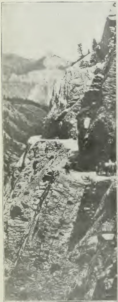
FIG. 1.—OURAY AND SILVERTON TOLL ROAD, COLORADO.
