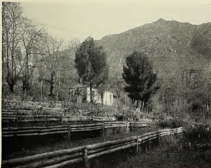
Temporary Office and Plant Nurseries, Kirstenbosch. A.C.S. Photo. July 20, 1914.
