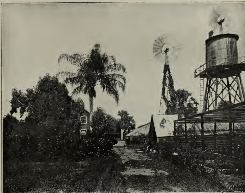
Water Tank, Greenhouses and Plant Packing House.
