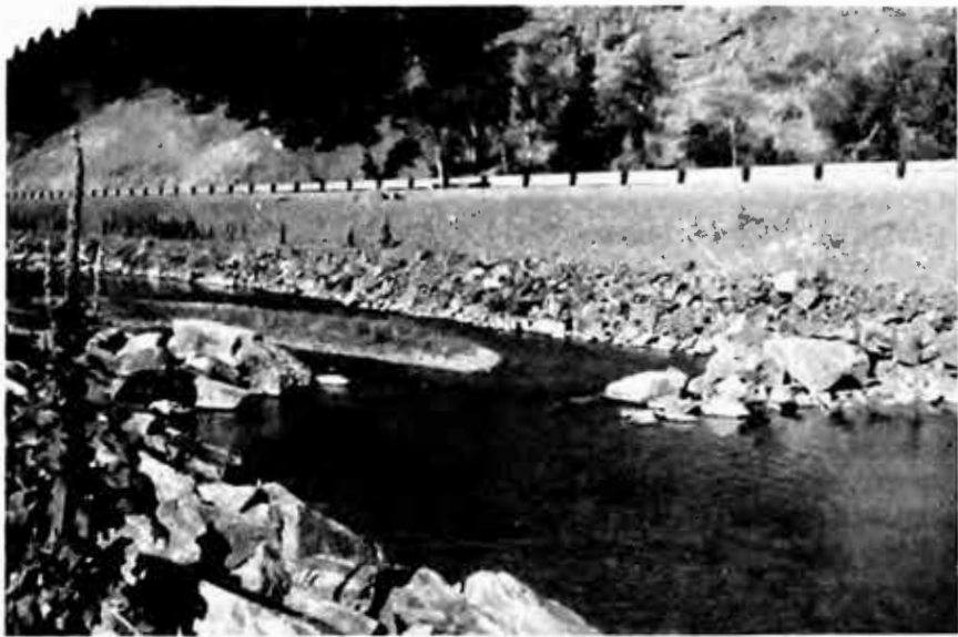
Rock jetties in altered stream channels were evaluated as habitat improvement structures by Montana Unit students.
