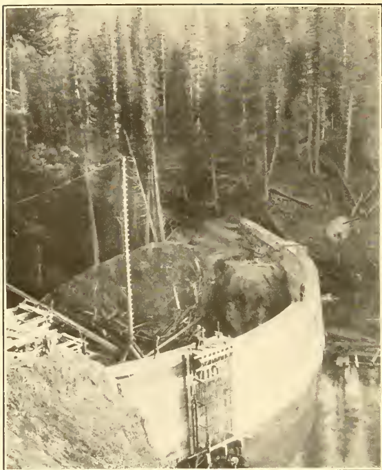
1. CLEAR CREEK DAM, TIETON UNIT OF YAKIMA PROJECT, WASHINGTON.
