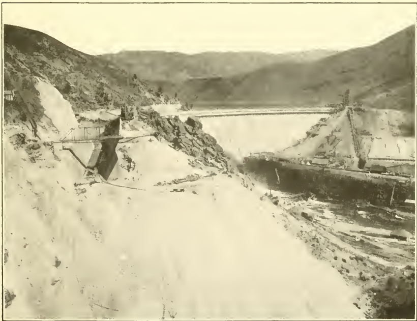
2. ARROWROCK DAM, BOISE RIVER, IDAHO. SPILLWAY CHANNEL ON THE LEFT.
