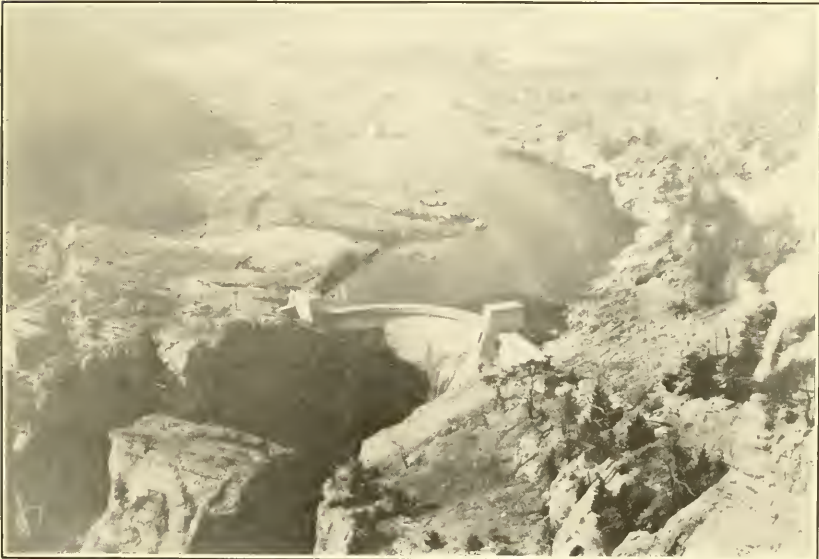
2. DIVERSION DAM IN SUN RIVER, MONT.
