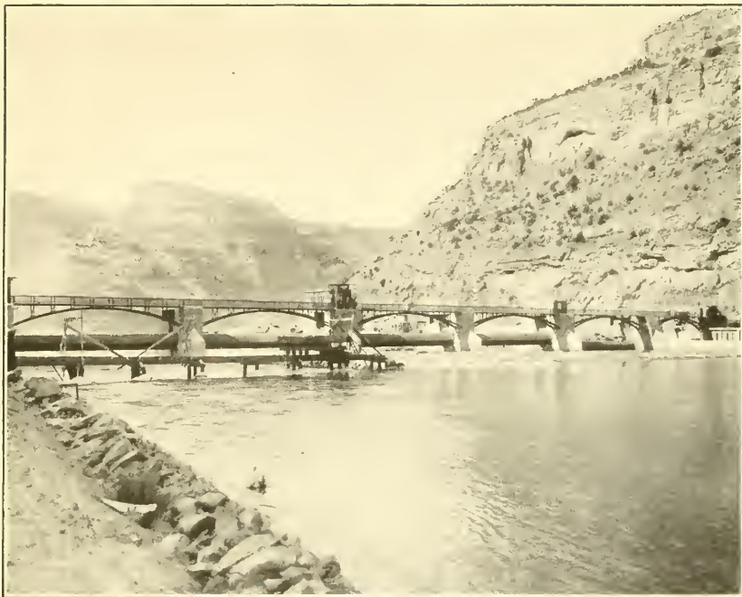
1. DIVERSION DAM, WITH ROLLER CRESTS IN GRAND RIVER, COLO.
