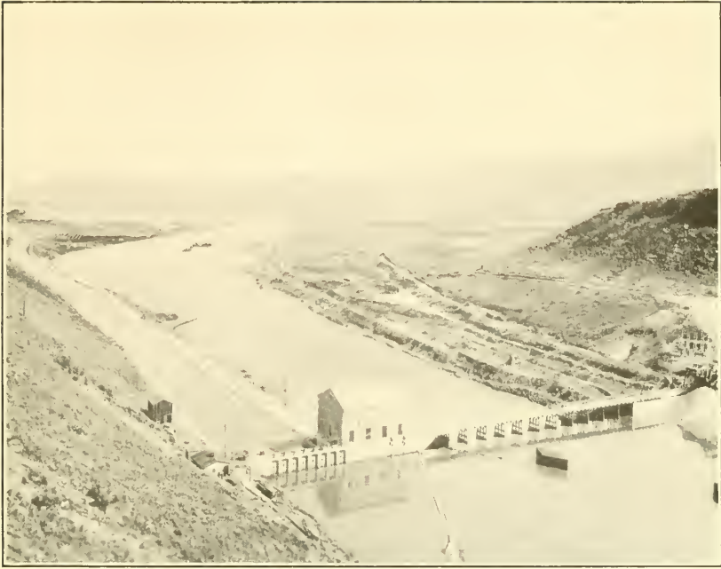
1. DIVERSION DAM IN BOISE RIVER, POWER PLANT AND HEAD OF MAIN CANAL.
