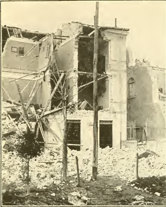
1.—RUINS OF AVEZZANO. THE REMAINS OF THE BANK OF NAPLES.
