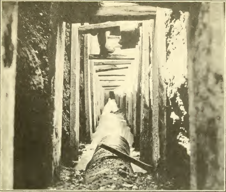
1. LAYING TILE DRAIN, HUNTLEY PROJECT, MONTANA.
