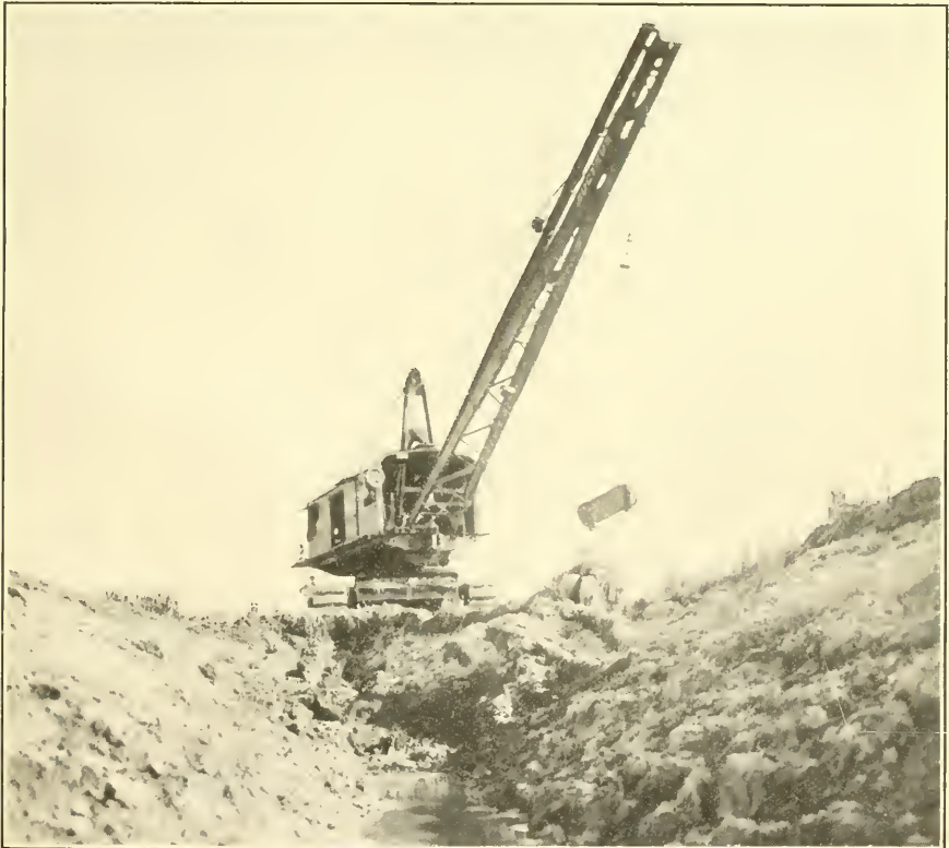
2. DRAGLINE EXCAVATING OPEN DRAIN DITCH, BOISE PROJECT, IDAHO.
