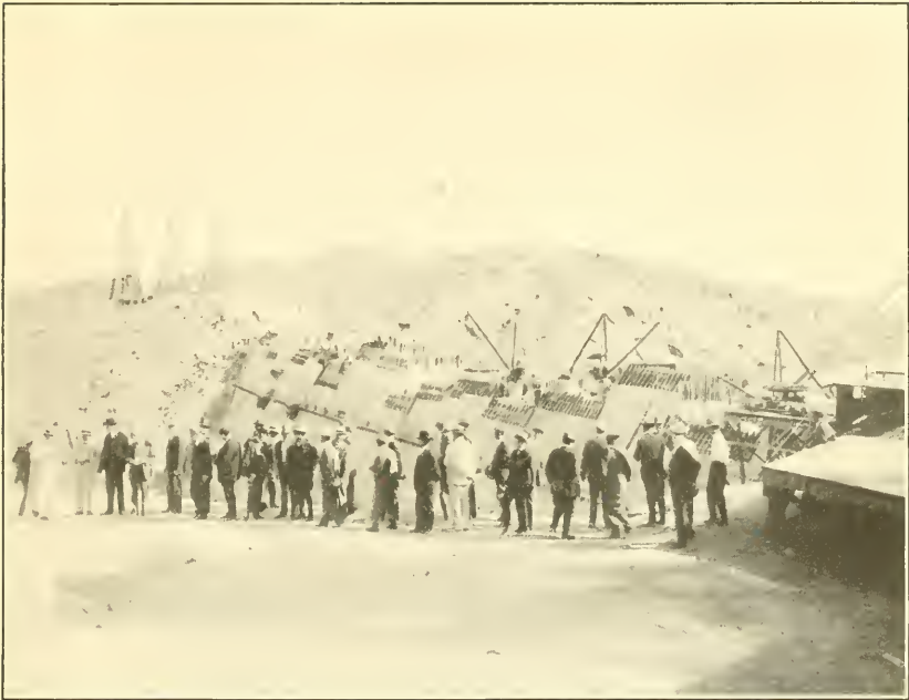
1. ELEPHANT BUTTE DAM IN THE RIO GRANDE, NEW MEX. CONGRESSIONAL PARTY ON TOUR OF INSPECTION, JUNE, 1915.
