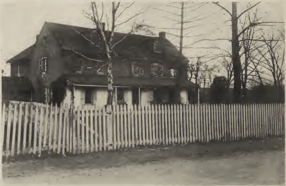
A HOUSE NEAR POTTSTOWN, PA., BEARING DATE 1804.
