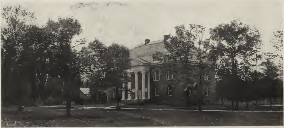
FIG. 11.—HALL OF SCIENCE, HAMILTON COLLEGE (1897). Clinton, N. Y. Carrère & Hastings, Architects.
