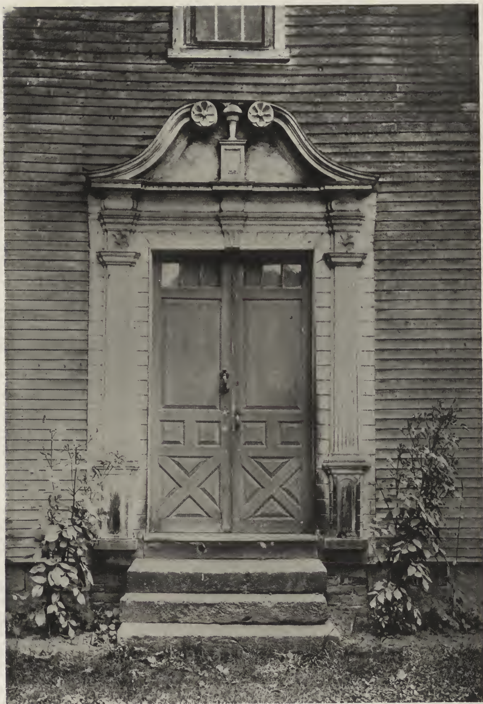
An ambitious Deerfield door which claims to have been built in 1750, the same year as the house, but is probably several decades later. It is a wooden copy of Georgian stone work even to the voussours. The broken pediment here used, became later a great favorite with Colonial builders and was much improved upon.
