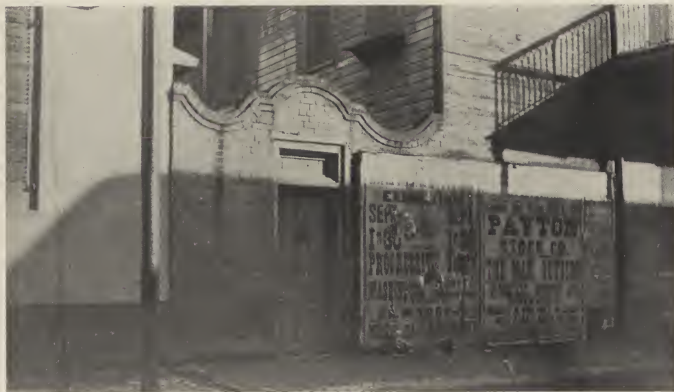
A COURTYARD ENTRANCE.
