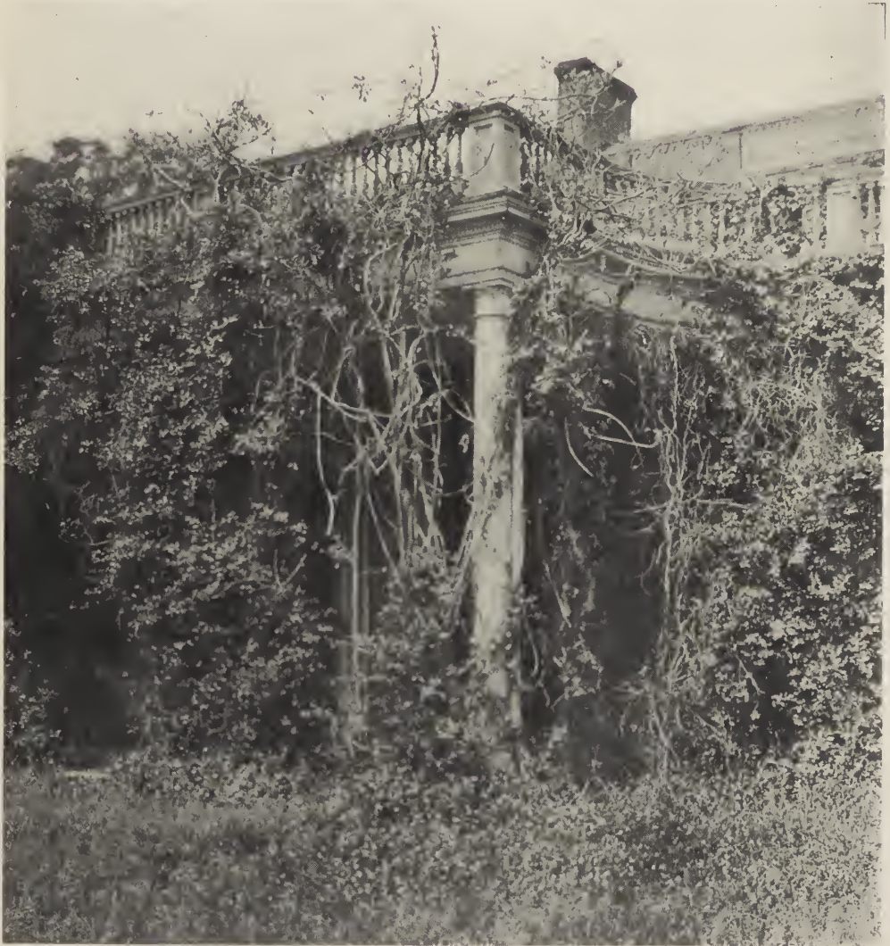
PORCH DETAIL, "MONTEBELLO." BALTIMORE, MARYLAND.
