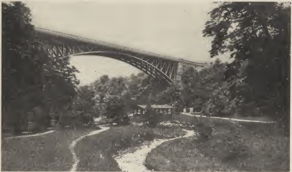
THE PANTHER HOLLOW BRIDGE.
