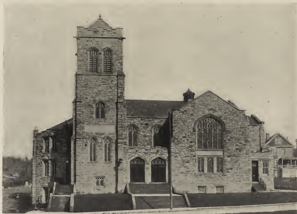
MARY S. BROWN MEMORIAL CHURCH. Geo. S. Orth & Bro., Architects.
