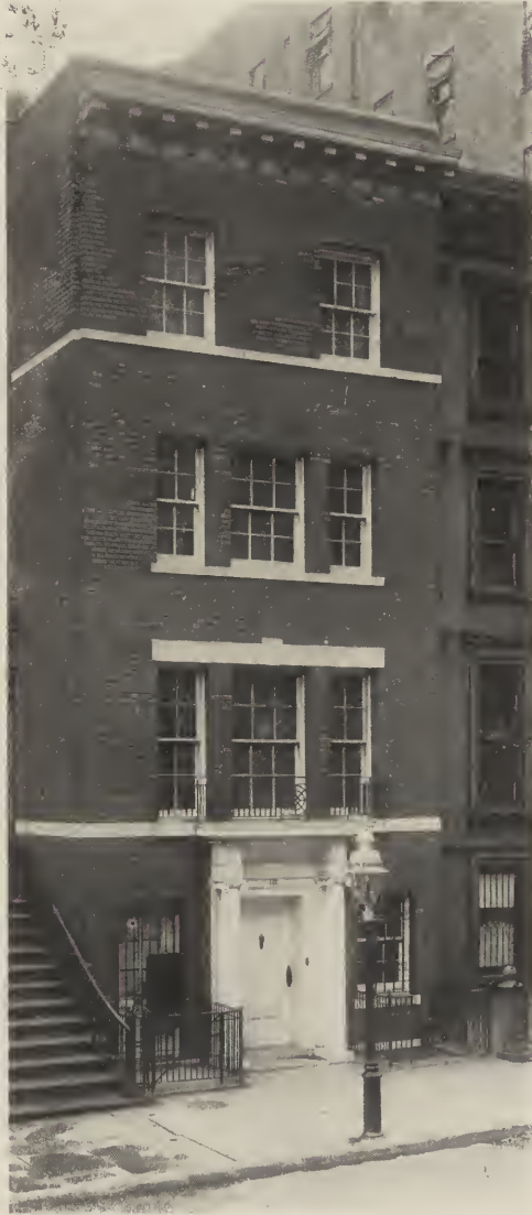
FIG. 11.—NO. 112 EAST 80TH STREET. Chas. E. Birge, Architect.
