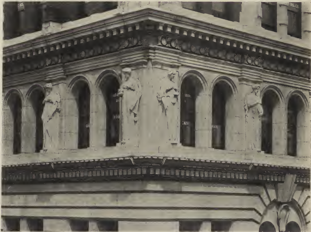
DETAIL OF THIRD STORY—FARMERS' BANK BUILDING.
