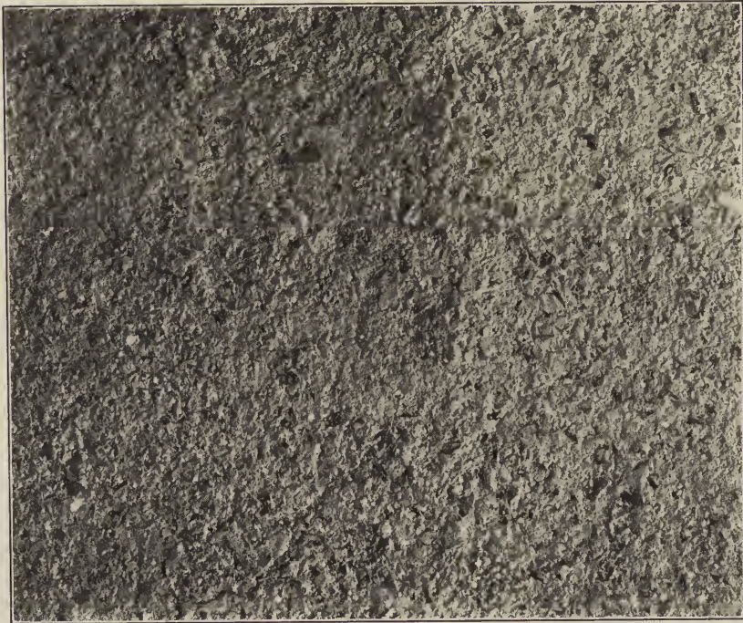
FIG. 8. SAND BLAST TREATMENT OF CONCRETE SURFACE.
