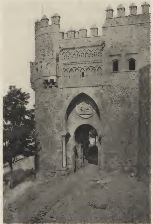
The Gate of the Sun, with Roman and Spanish Stone Work, Mudejar Brick Work, and Visigothic Columns.
