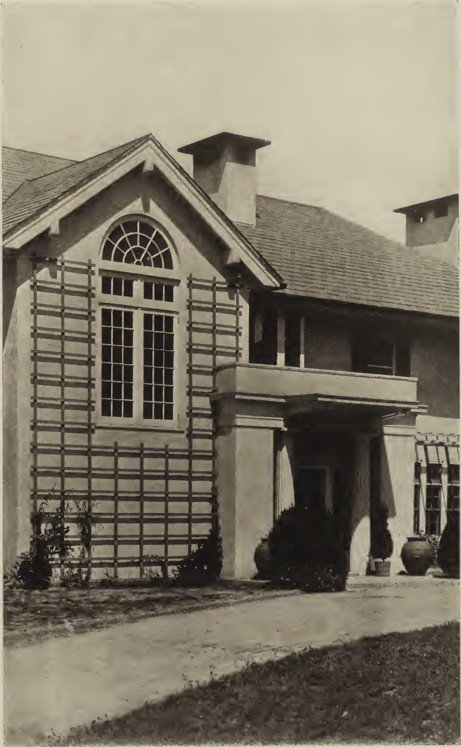
ENTRANCE DETAIL. RESIDENCE OF J. N. TILDEN, ESQ. MANITOU, N. Y. ALBRO AND LINDBERG, ARCHITECTS.
