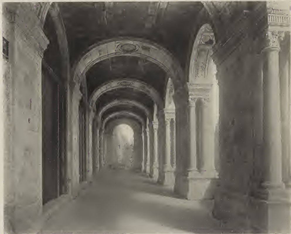
LOGGIA DETAIL—THE HERMITAGE HOTEL.
