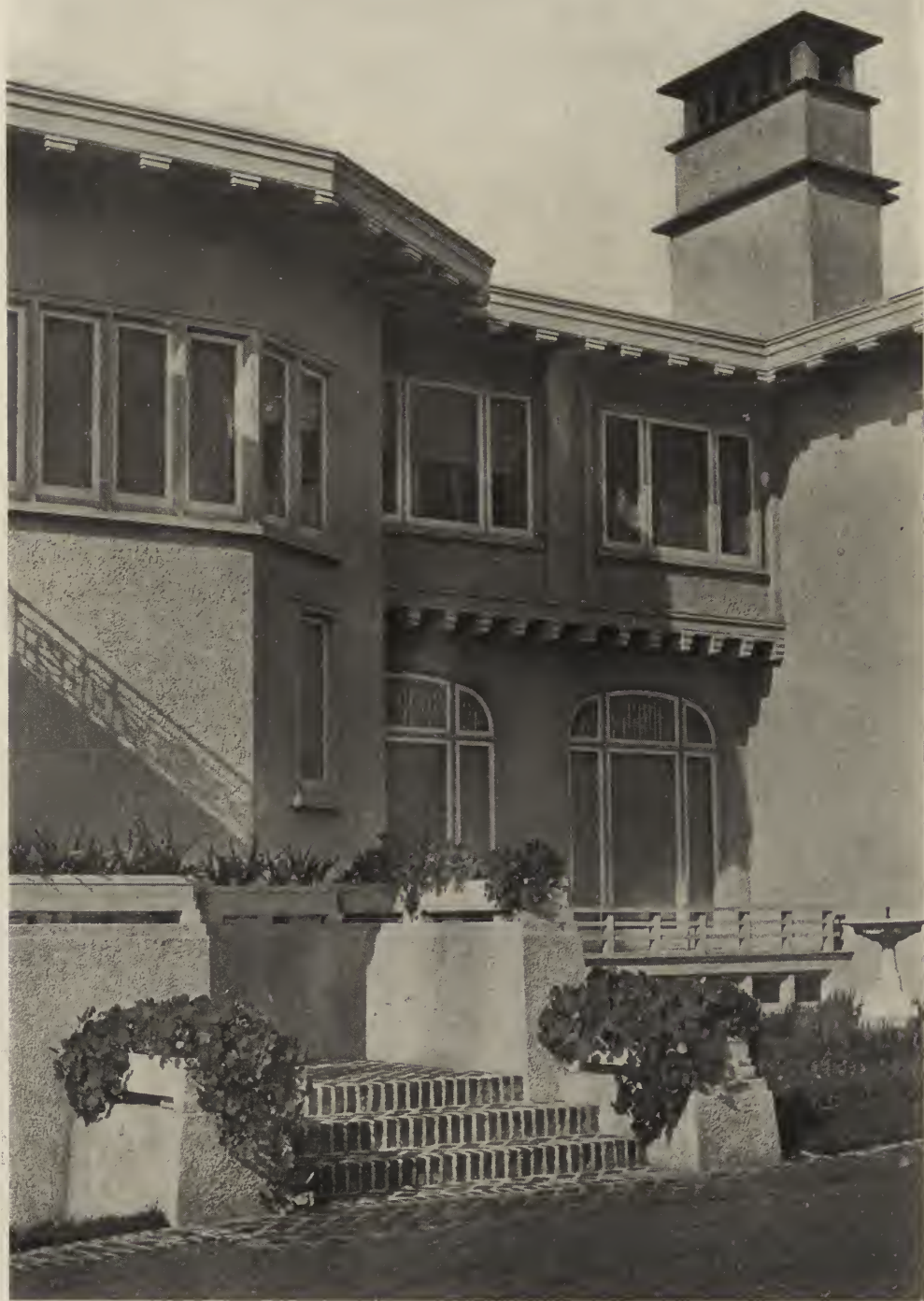
DETAIL—RESIDENCE OF MRS. JAMES MOFFITT, PIEDMONT PARK, CAL. LOUIS C. MULLGARDT, ARCHITECT.
