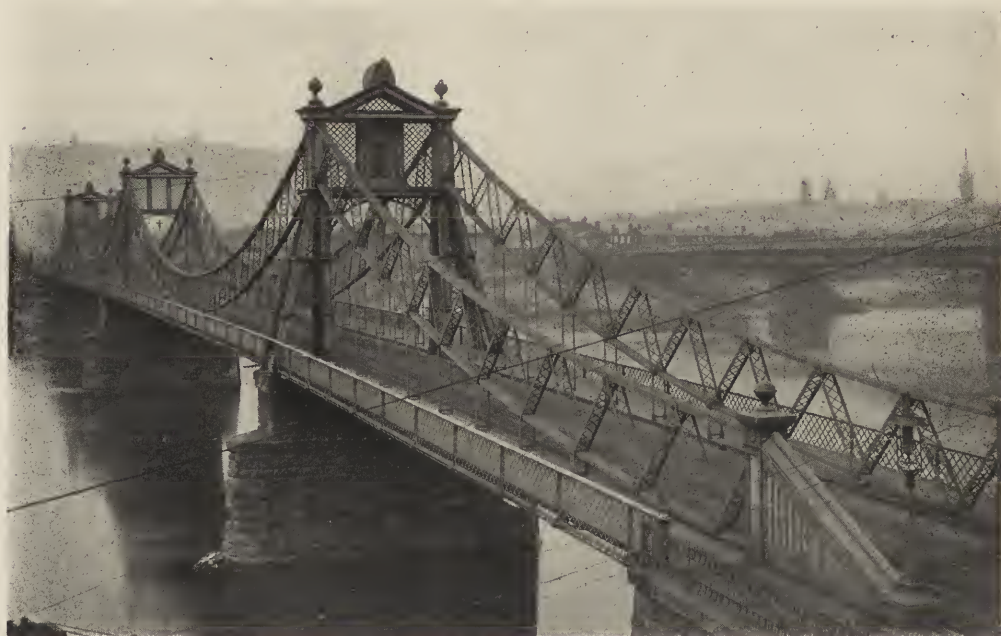
THE SEVENTH STREET BRIDGE, PITTSBURGH, PA. Gustav Lindenthal, Engineer.
