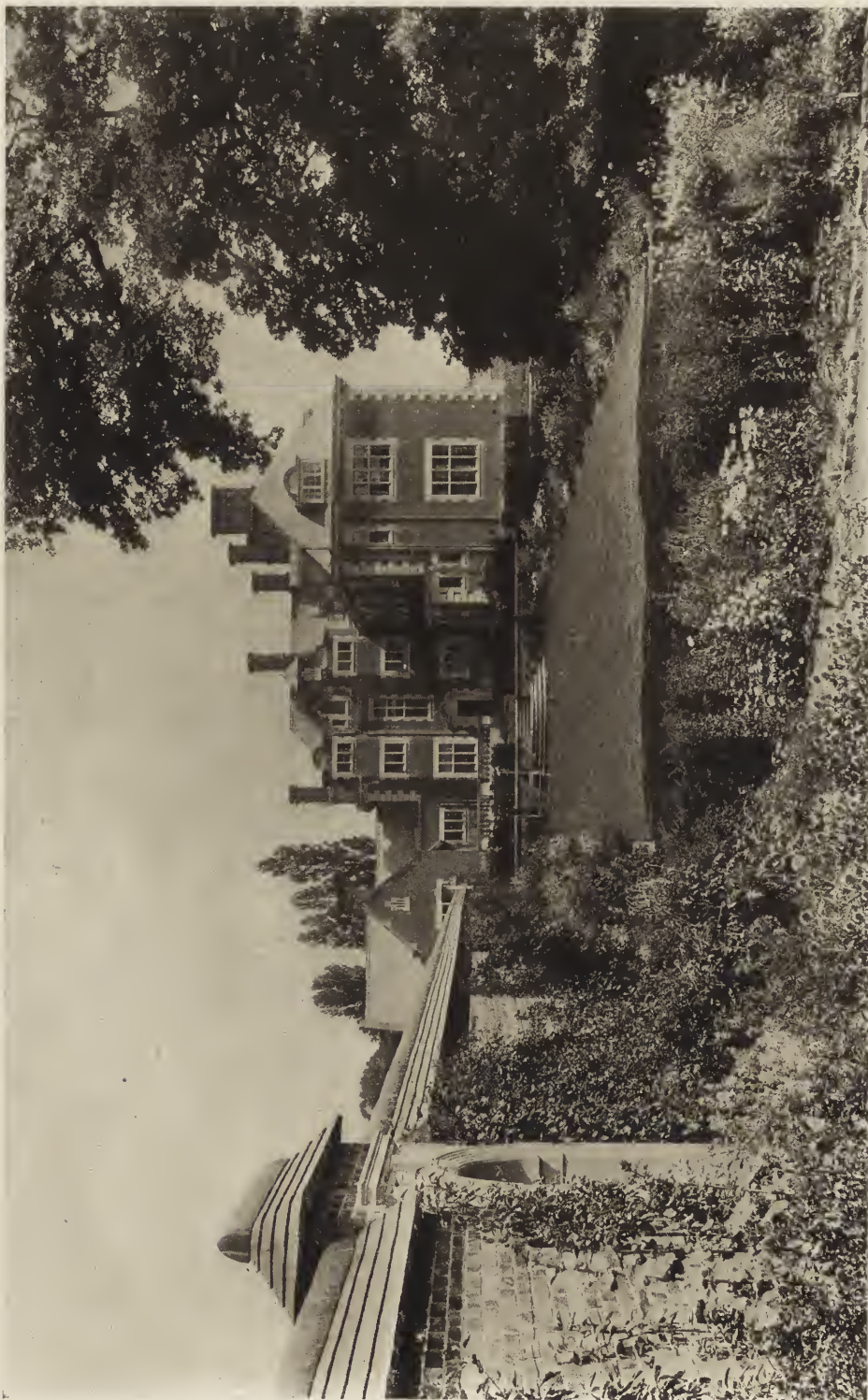
GARDEN WALL AND CROQUET LAWNS AT DUNCHURCH LODGE, RUGBY. Gilbert Fraser and Thomas H. Mawson, Associate Architects.
