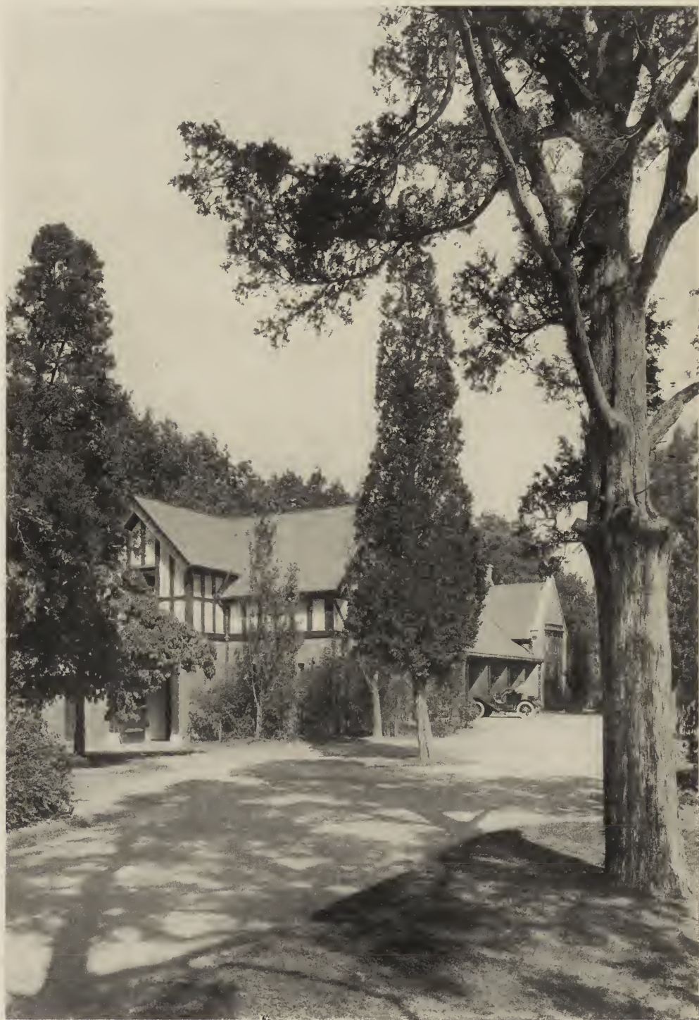
GARAGE—W. J. MATHESON, ESQ. Fort Hill, L. L. Clinton Mackenzie, Arch't.
