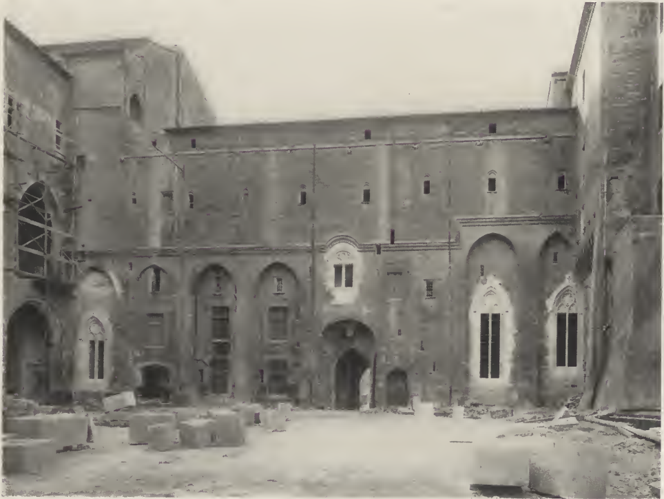
WESTERN FAÇADE FACING COURTYARD.
