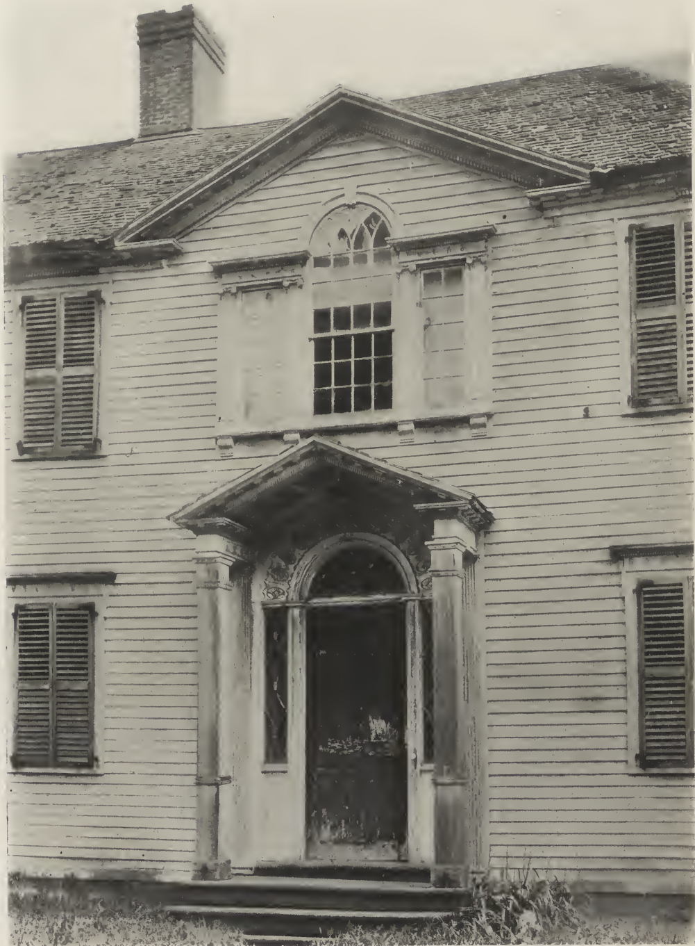
One of the most extraordinary things about this excellent piece of work is that it was found in a very small unknown Connecticut town called Bethany. The carved frieze over the arch is unique, in no sense typical of Colonial. Cornice and carved panels of the soffit of the hood are well executed as to suggest that the coarser boxed posts of the porch probably replace original columns. The Palladian motif above the door is full of quality.
