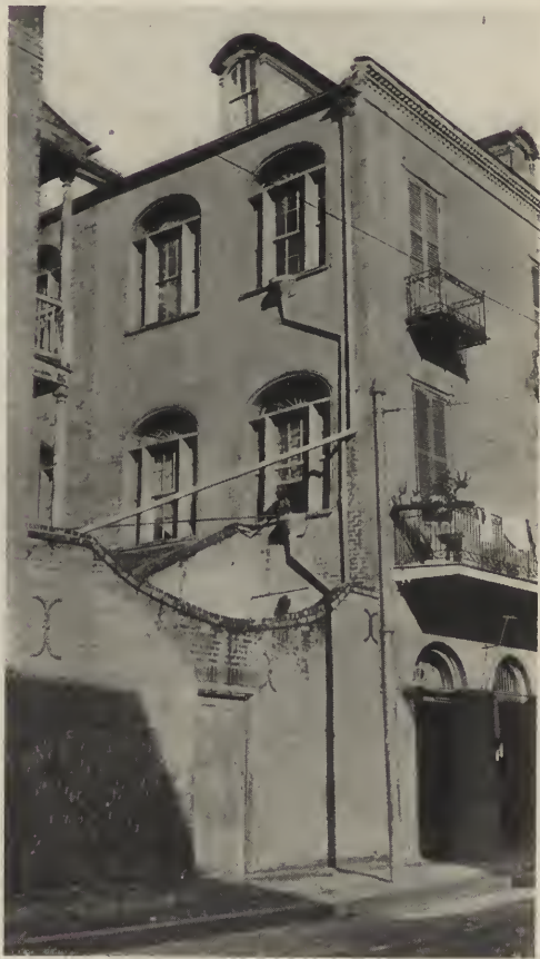
A COURTYARD ENTRANCE.
