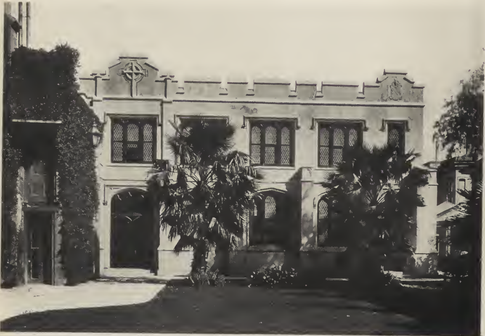
HOWCOTT MEMORIAL—TRINITY PARISH HOUSE.
