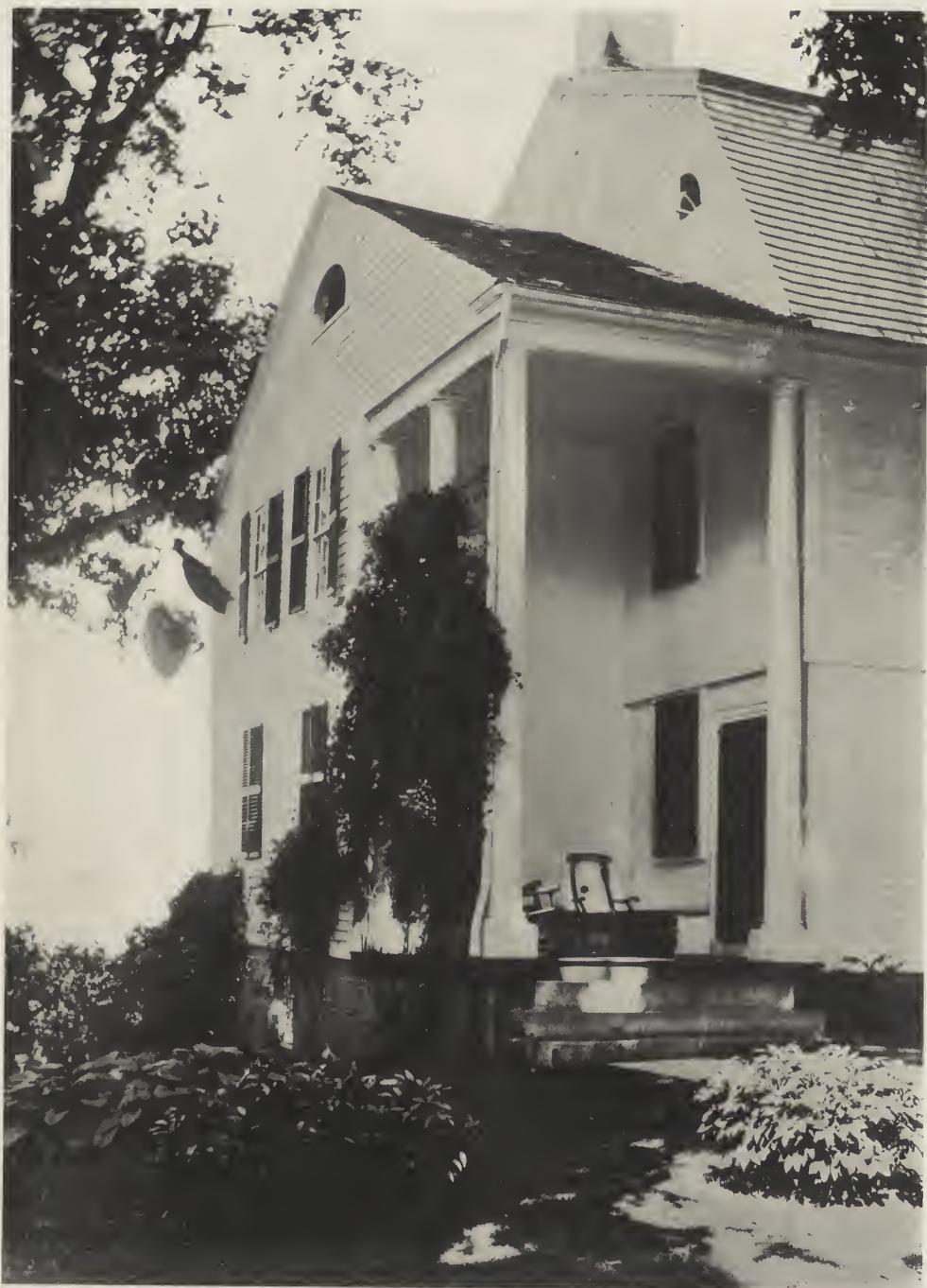
An unexcelled end treatment of a house and incidently of a doorway. It is in Litchfield and tradition has it that its owner, before building it, had visited Mt. Vernon. Vignola has been absolutely disregarded in proportioning the columns and the resulting delicacy is peculiarly appropriate to wood. The other end of the house has the same motif.
