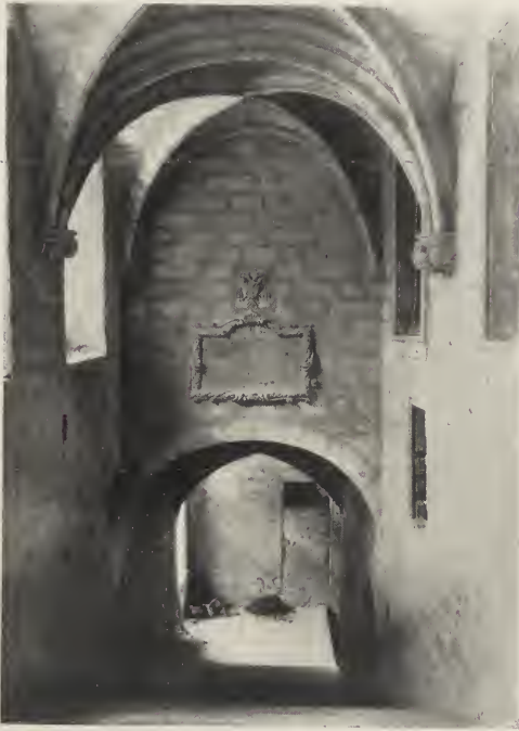
STAIRCASE LEADING TO THE PONTIFICAL CHAPEL OF CLEMENT VII—RESTORED IN 1659.
