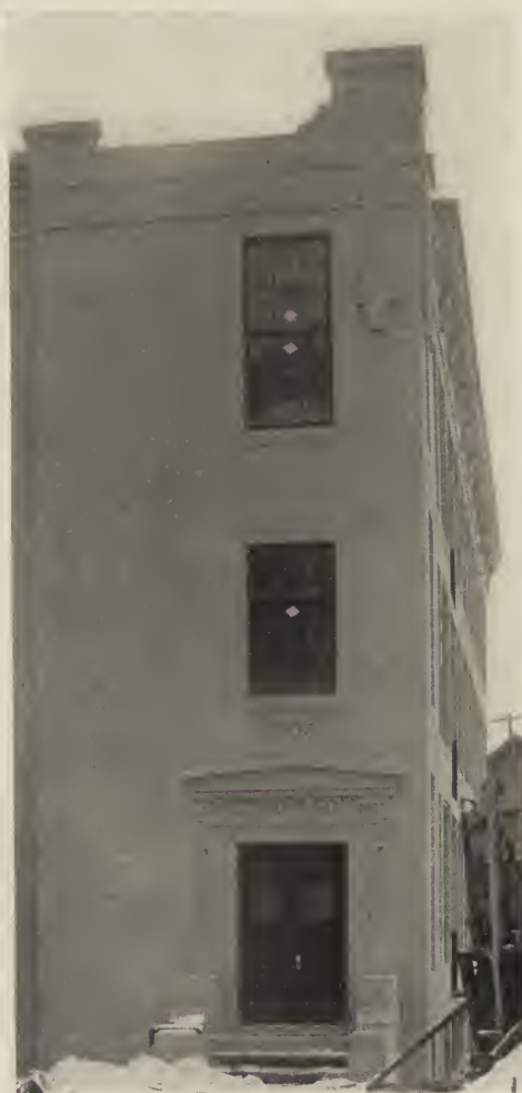
FIG. 6. SKILFUL TREATMENT OF A CONCRETE CORNICE.
