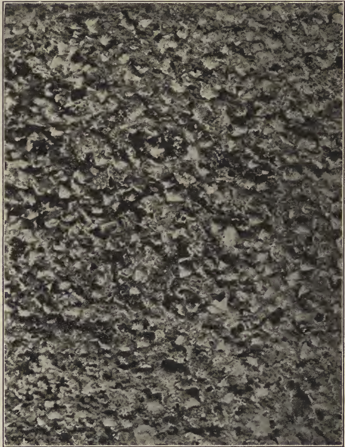
FIG. 10. SURFACE FINISHED BY PNEUMATIC HAMMER.
