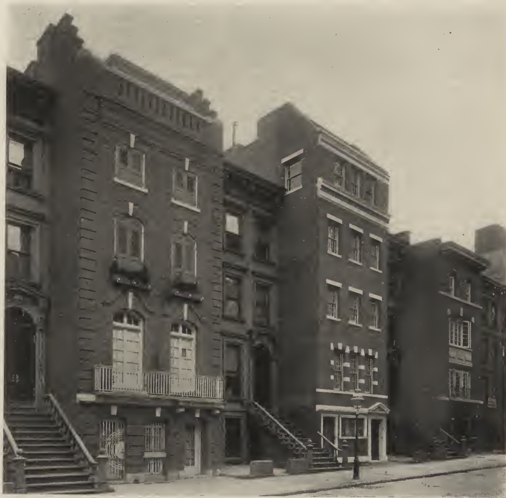
FIG. 13.—NOS. 122-126-130 EAST 80TH STREET. Schwartz & Gross, Architect.
