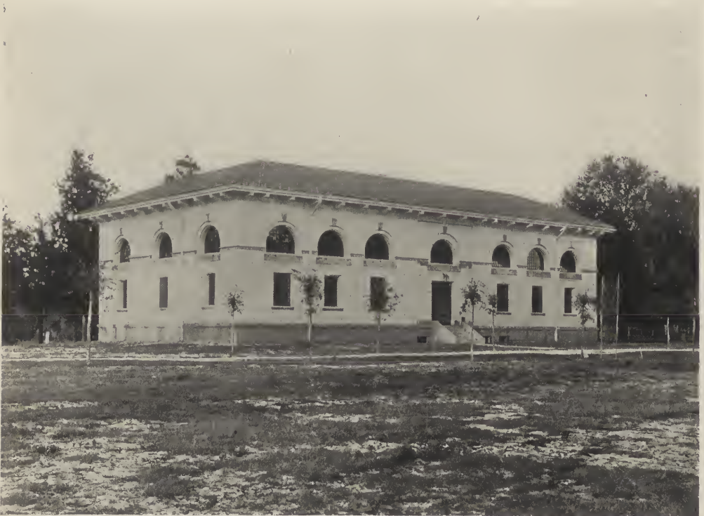
LIBRARY AND ADMINISTRATION BUILDING—ROLLINS COLLEGE.
