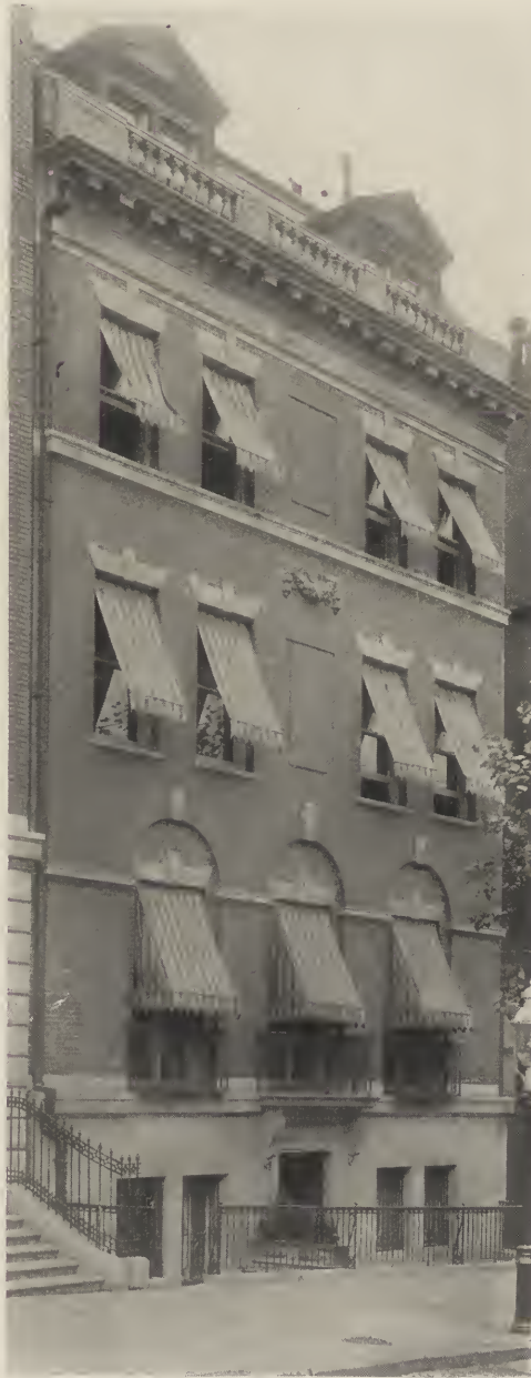
FIG. 9.—754 PARK AVENUE. Geo. H. De Gersdorff, Architect.
