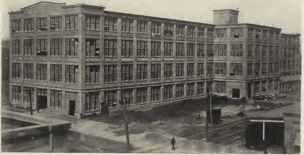
FIG. 4. A REINFORCED CONCRETE FACTORY BUILDING.
