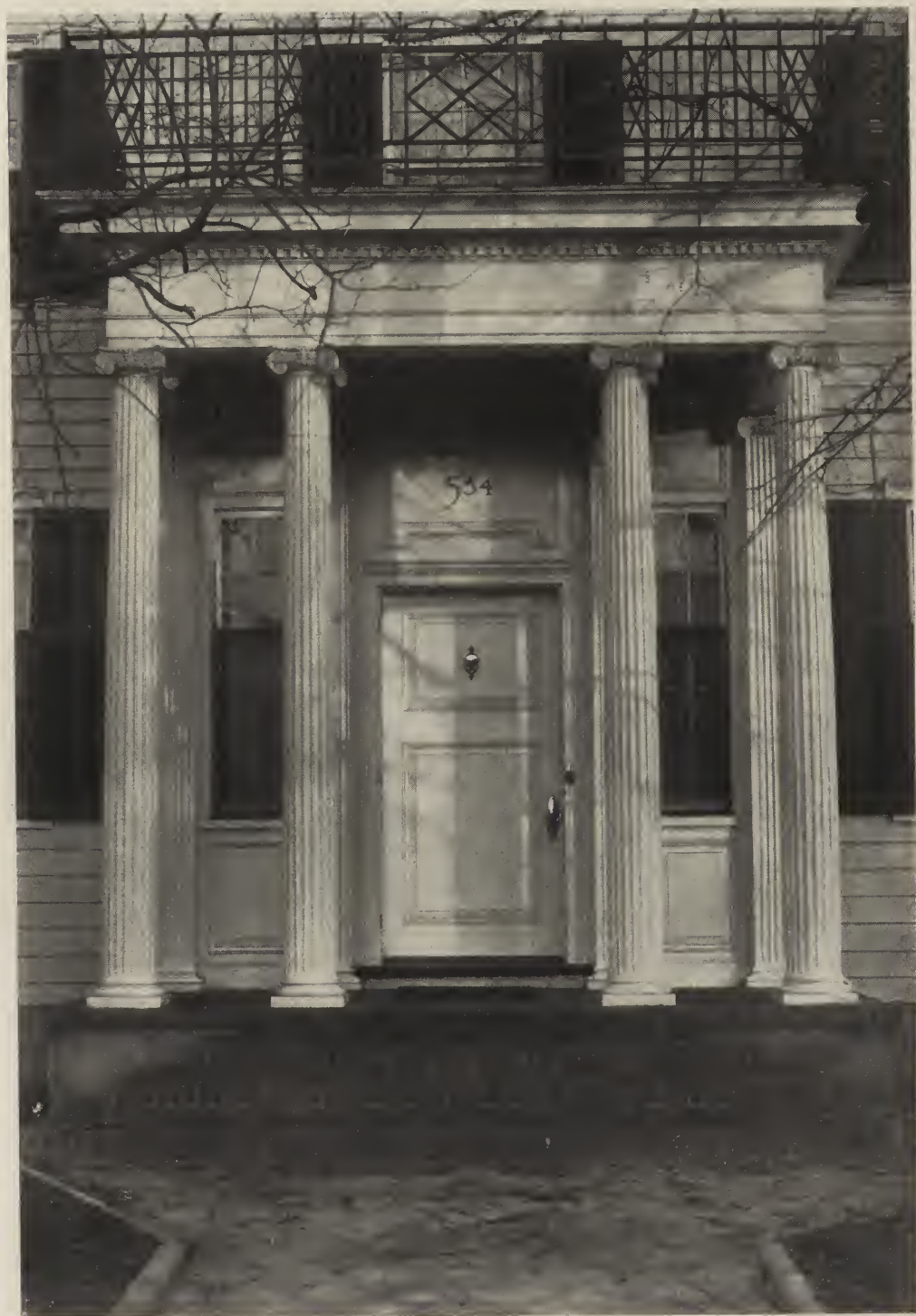
DETAIL OF ENTRANCE PORCH—RESIDENCE OF W. P. COLEMAN, ESQ., MACON, GA. Hentz & Reid, Architects.
