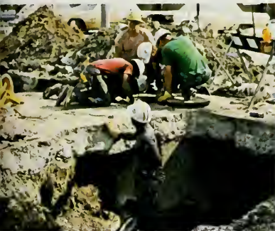
... of Pennsylvania crew turns attention to ... water-logged underground cable.
