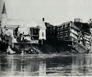
... Ellsville, New York church and hospital undermined ... by flooding Genesee River.
