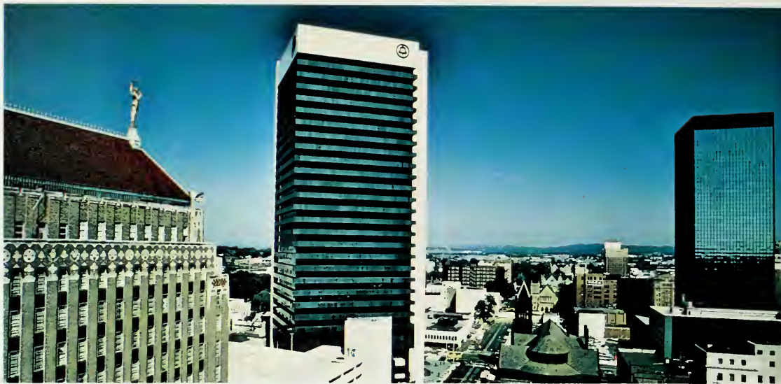
SCB, Birmingham, headquarters.
