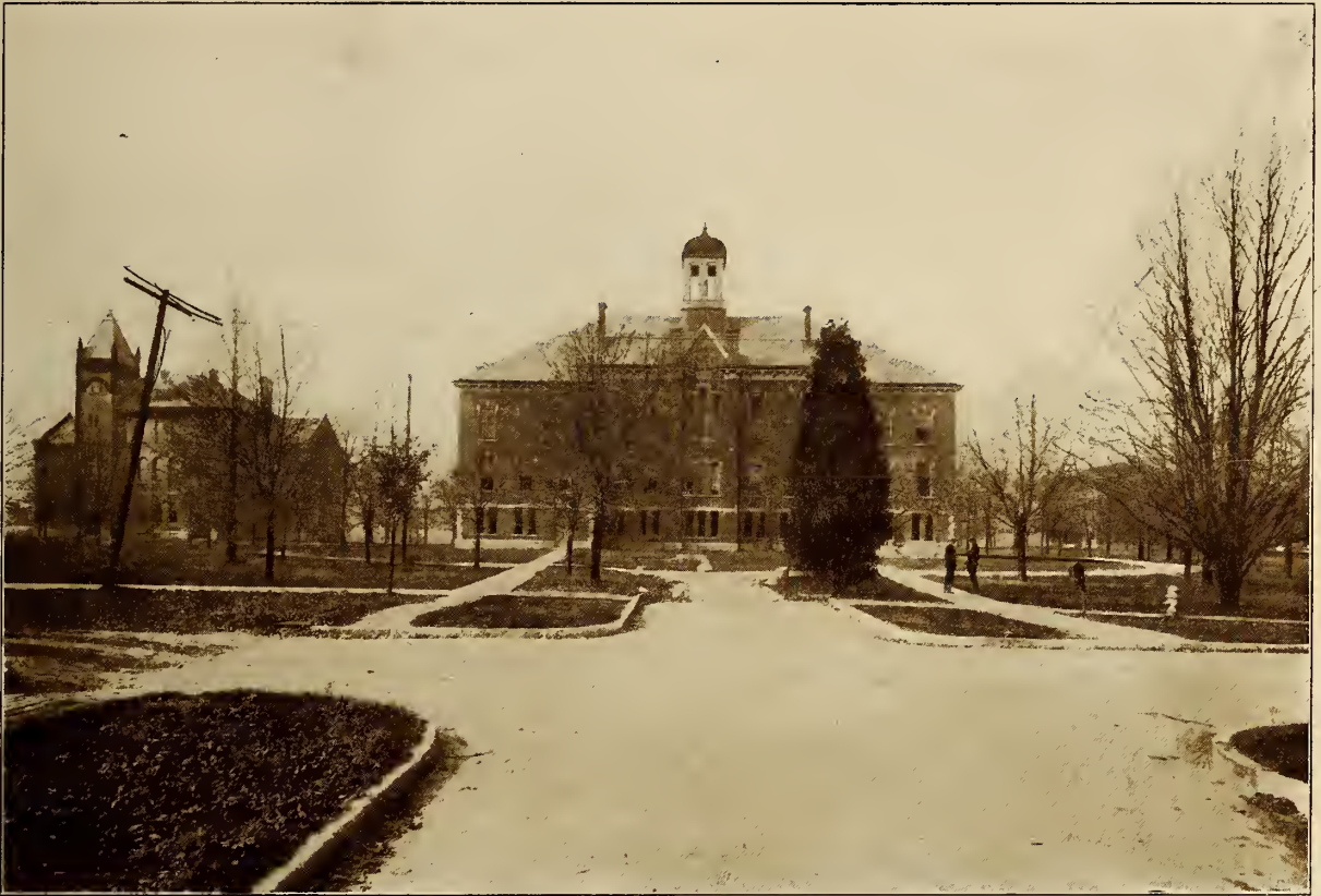
Main Approach, From University Avenue
