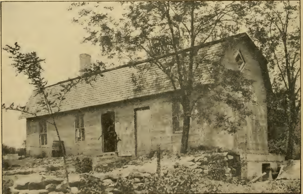
David Running's 16 x 40-foot concrete building. The end view of this building and the entrance to the bee-cellar are shown on our cover.
