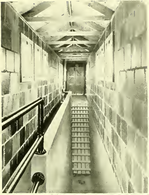
Dipping Vat U.S. Army Remount Station Front Royal
