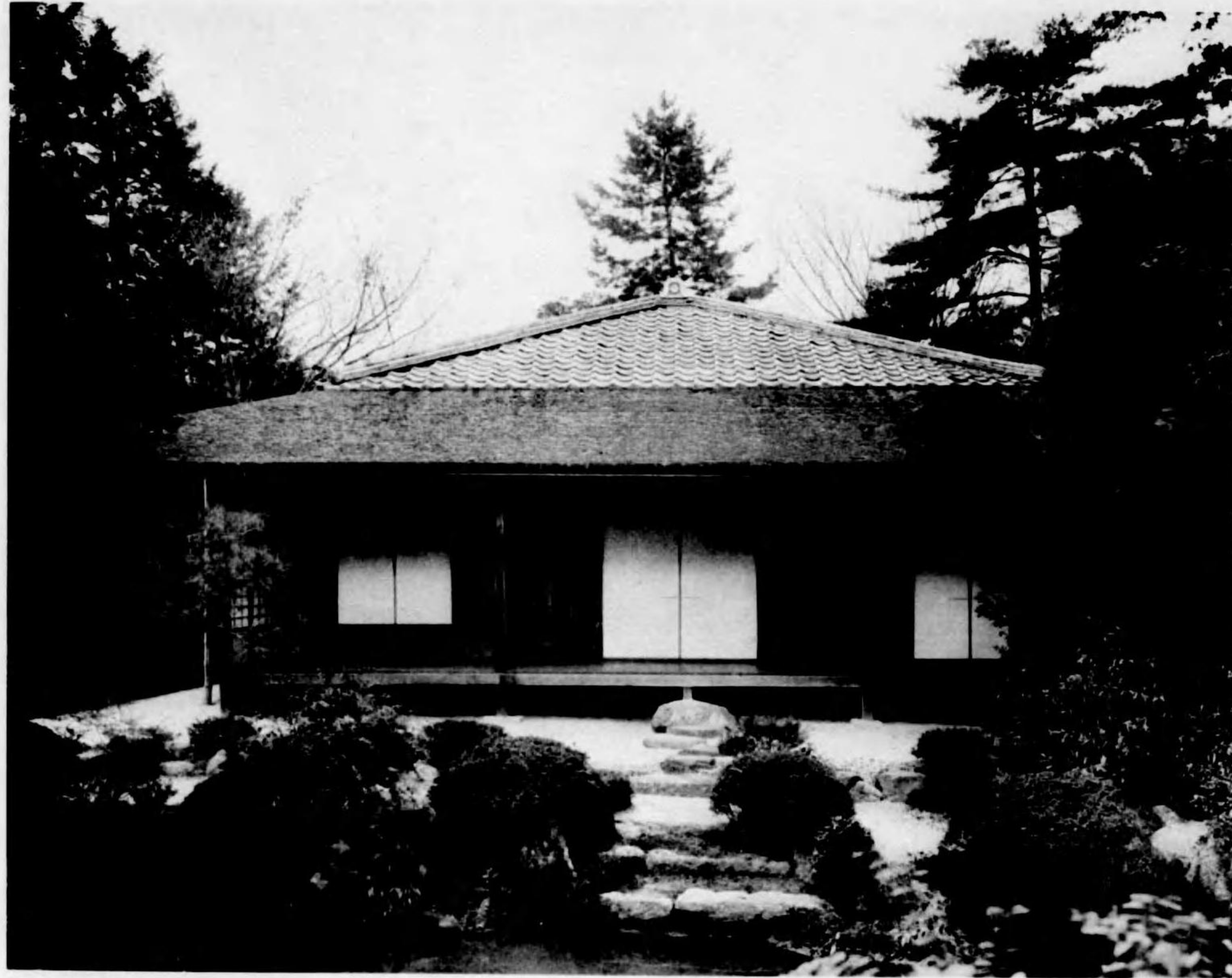
神學院書院 中ノ御茶屋 御茶屋 御茶屋 South side view of Residence , Middle villa, Shogun in Detached Palace.
