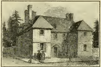
PENN'S HOUSE IN PHILADELPHIA Built of English brick and roofed with slate.
