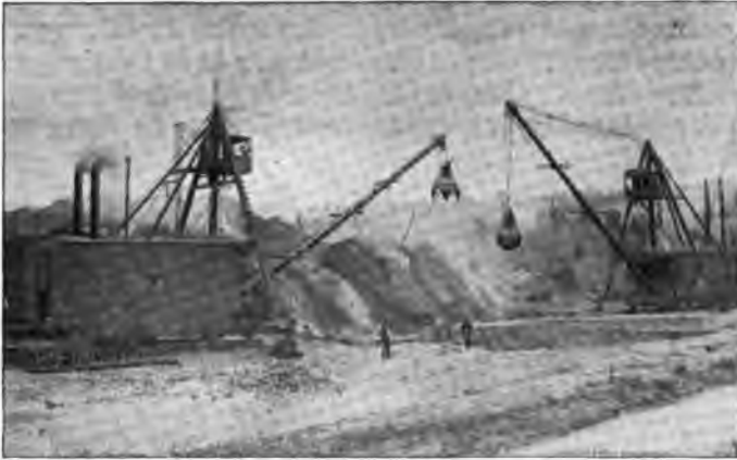
WORKING LOW GROUND BY DREDGE.
